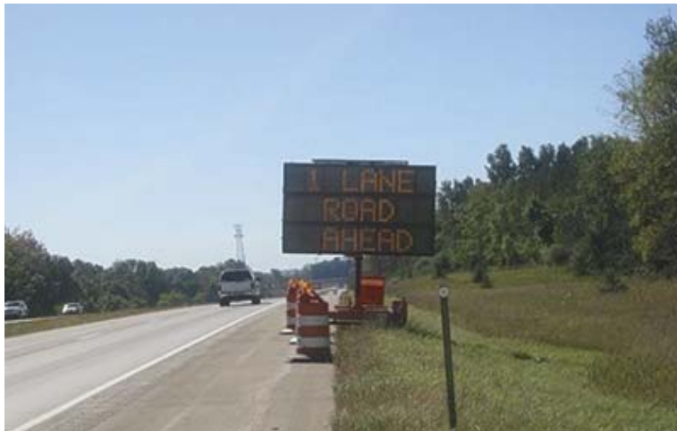
Figure 2.3 Portable dynamic message sign (Scriba & Seplow 2006)
