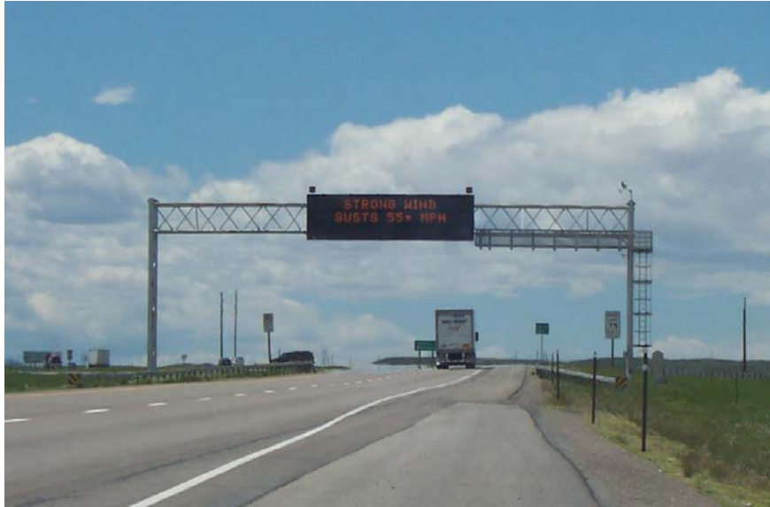
Figure 3.3 Three-line Overhead DMS at milepost 356.7, westbound
