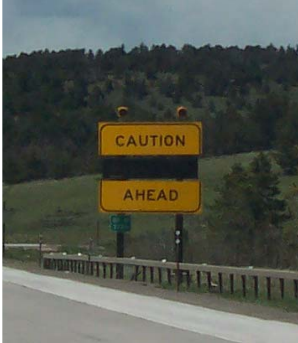
Figure 3.4 One-line Blank-Out DMS at milepost 322.6, westbound
