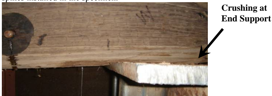
Figure 5.4 Crushing at west end support of Specimen 1
