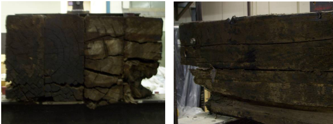
Figure 3.1 Deterioration and damage for Specimen 3 (left: splits on the end; right: longitudinal cracks)
