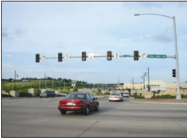
Figure 1.2 Cantilever Traffic Signal and High-Mast Luminaire
