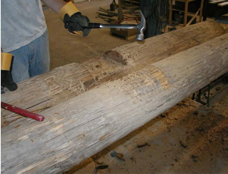
**Figure 3.6** Breaking the Fingers Out of the Notch with a Hammer
