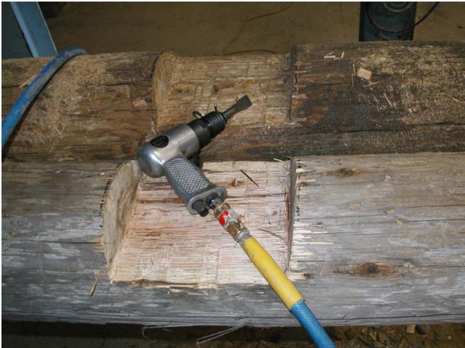
**Figure 3.7** The Finished Notch After Using the Air Chisel
