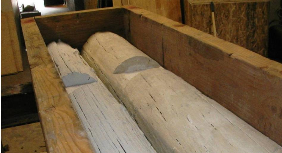
**Figure 3.14** View Inside the Form Before the Rebar is Installed
