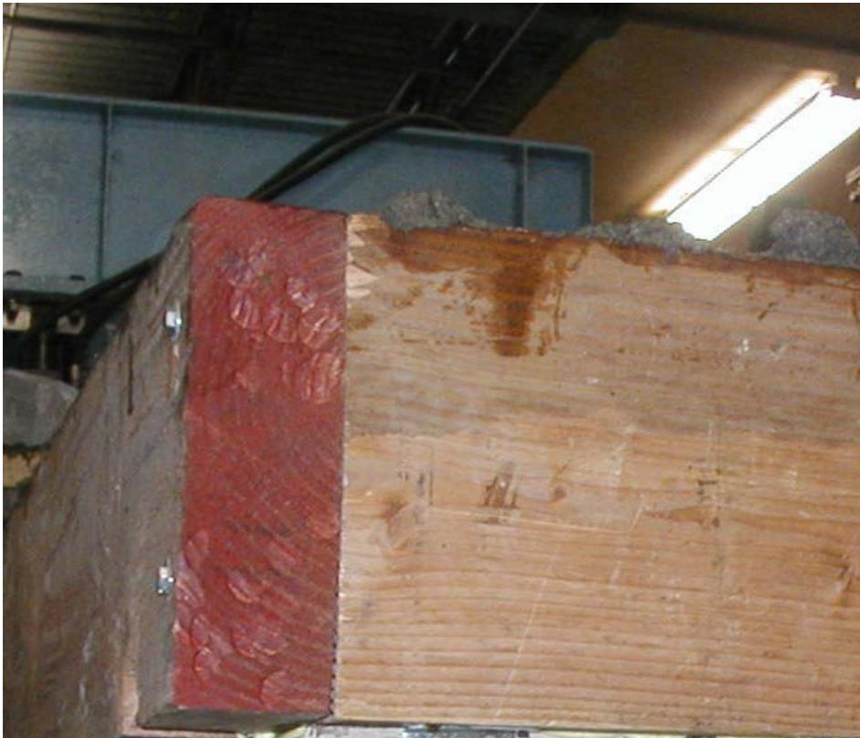
**Figure 3.11** Lag Bolts at the Corner of the Formwork
