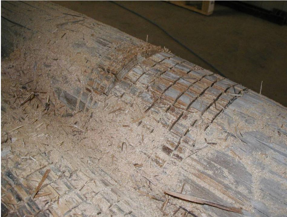
**Figure 3.5** Cutting the Shear Key Notch for the Connection
