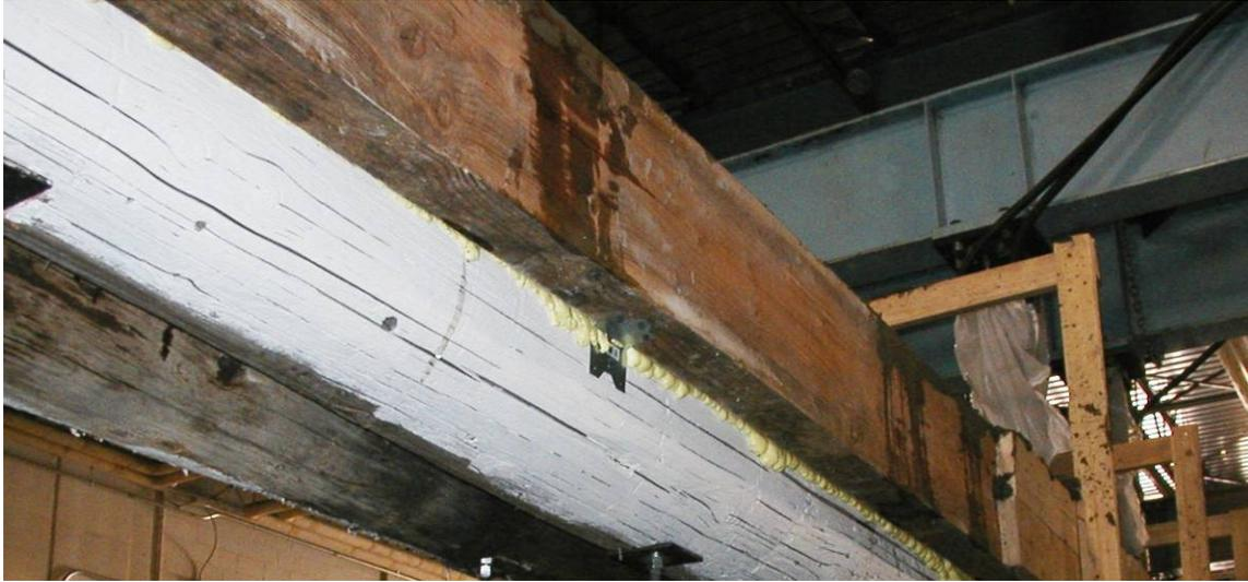
**Figure 3.18** Bottom of the Formwork Showing the Foam Gap Filler
