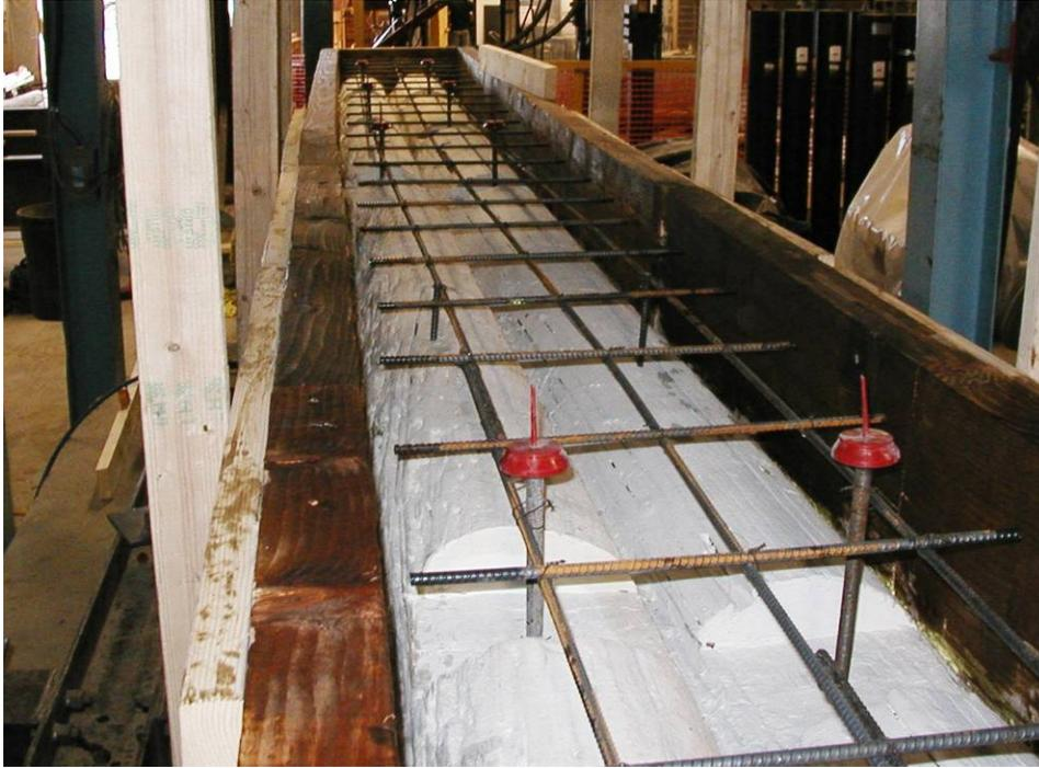
**Figure 3.17** Rebar Layout
