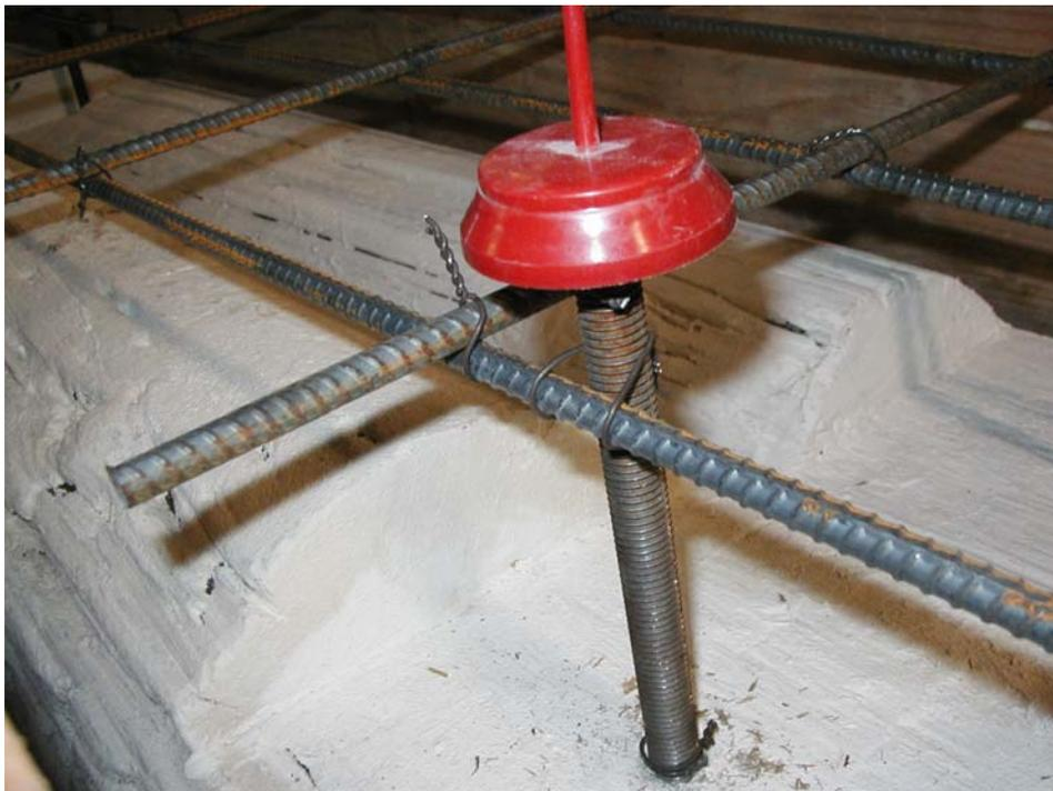
**Figure 3.16** Rebar Tie Wire Loop to Hold the Threaded Rod
