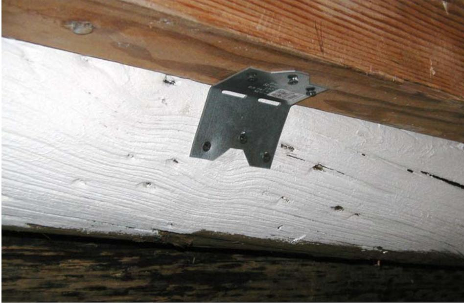
**Figure 3.12** Simpson Angle Bracket Model LS30
