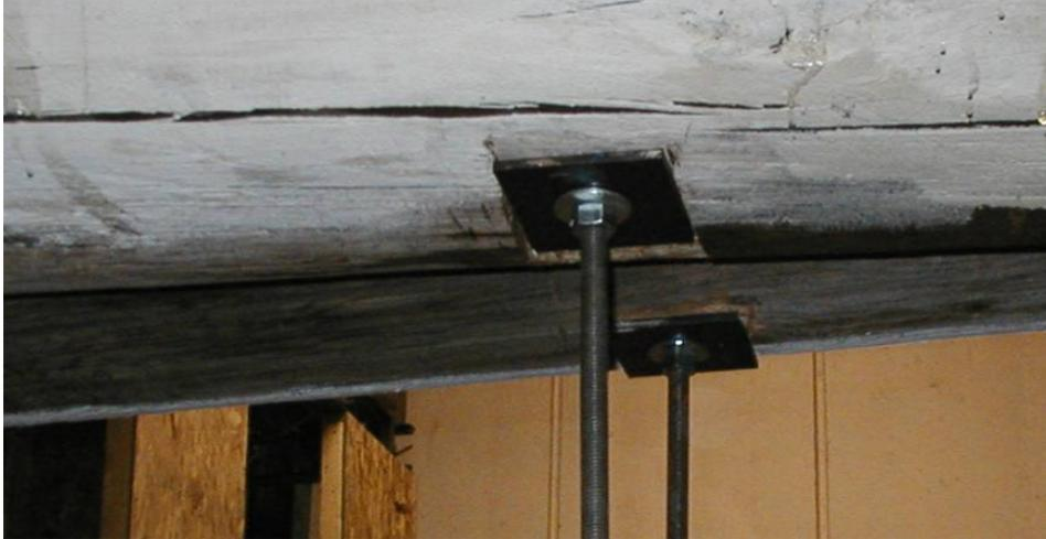
**Figure 3.15** Bearing Plate Assembly
