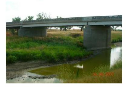
**Figure 4.4** Moreau River Bridge near Faith (from left bank facing along downstream face toward right bank). The pier sets in the picture are bent 5 (left) and 4 (right).
