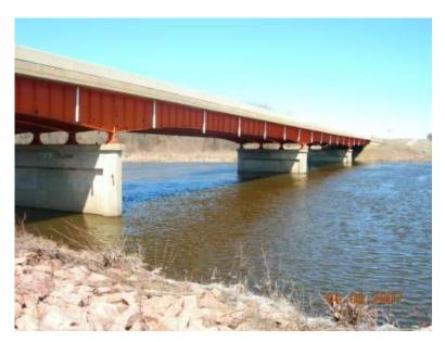
**Figure 4.3** Big Sioux River Bridge near Flandreau (from left bank facing along upstream face toward right bank). The pier sets in the picture are, from left to right, bent 4, 3, and 2.
