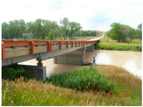
**Figure 9.3** Picture from left bank facing along upstream face toward right bank. The two main channel piers are bent 2 (adjacent to left bank) and bent 3 (adjacent to right bank).
