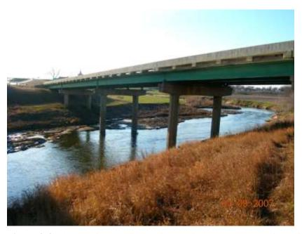
**Figure 8.4** Picture of bridge from left bank facing downstream face of the westbound bridge. Bent 3 is the pier set in the low-flow channel. The two adjacent pier sets are bent 2 (right bank) and bent 4 (left bank).
