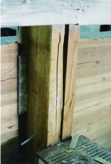
Figure 28 Vertical split in false work post
