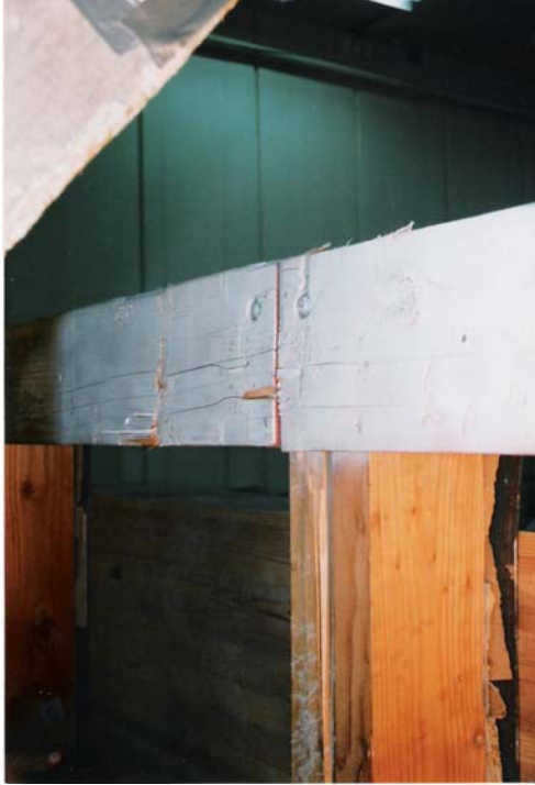
Figure 25 Bearing indentation in rail
