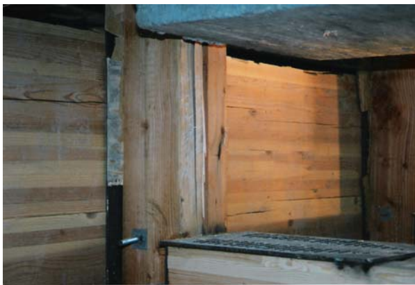
Figure 21 Horizontal cracks in through girder
