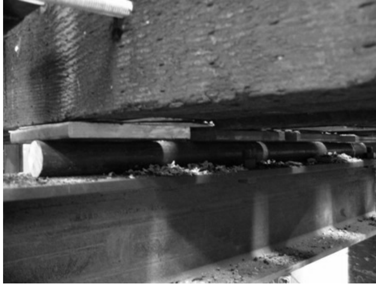
Figure 4.4: Timber stringer on steel crossbeam, round stock, and plates
