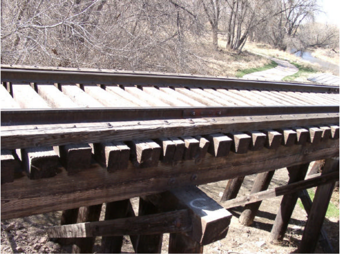
Figure 2. Standard open-deck timber trestle railroad bridge
