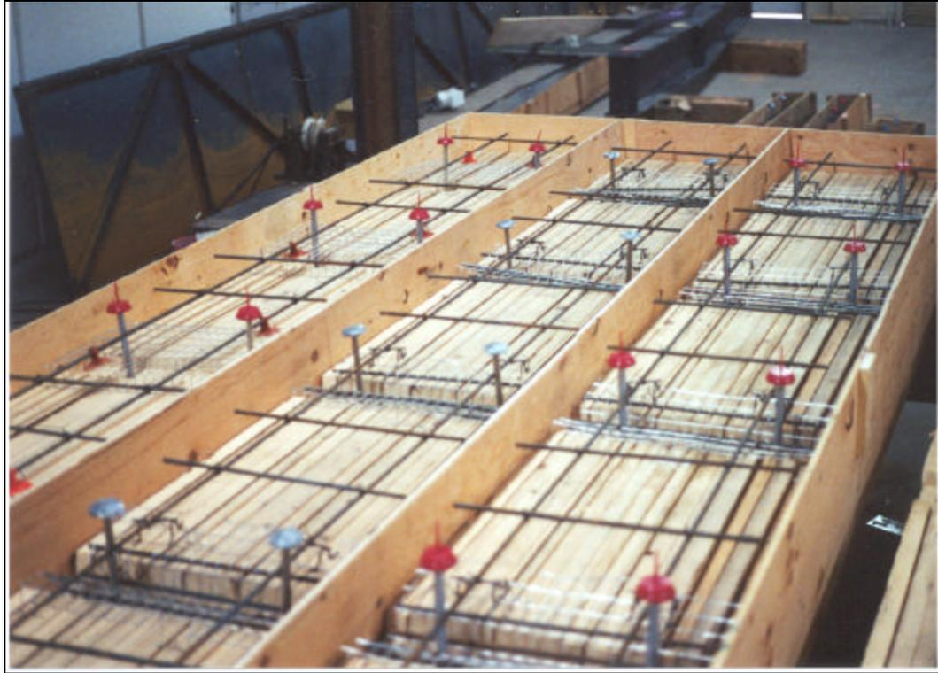
**Figure 3.15 Rebar Placement for Beams 3 and 4**
