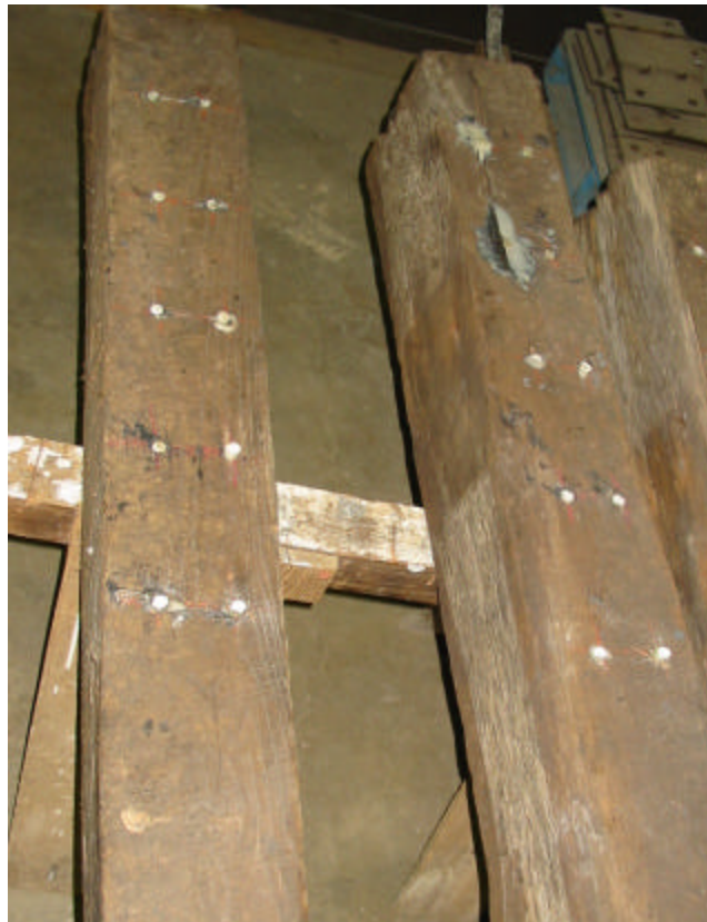
Figure 6. Crossties with shear spikes installed
