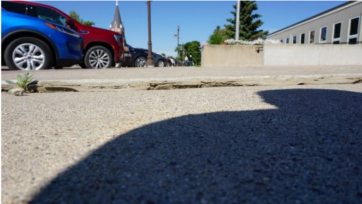
Figure 20. Sidewalk displacement along Third Street
