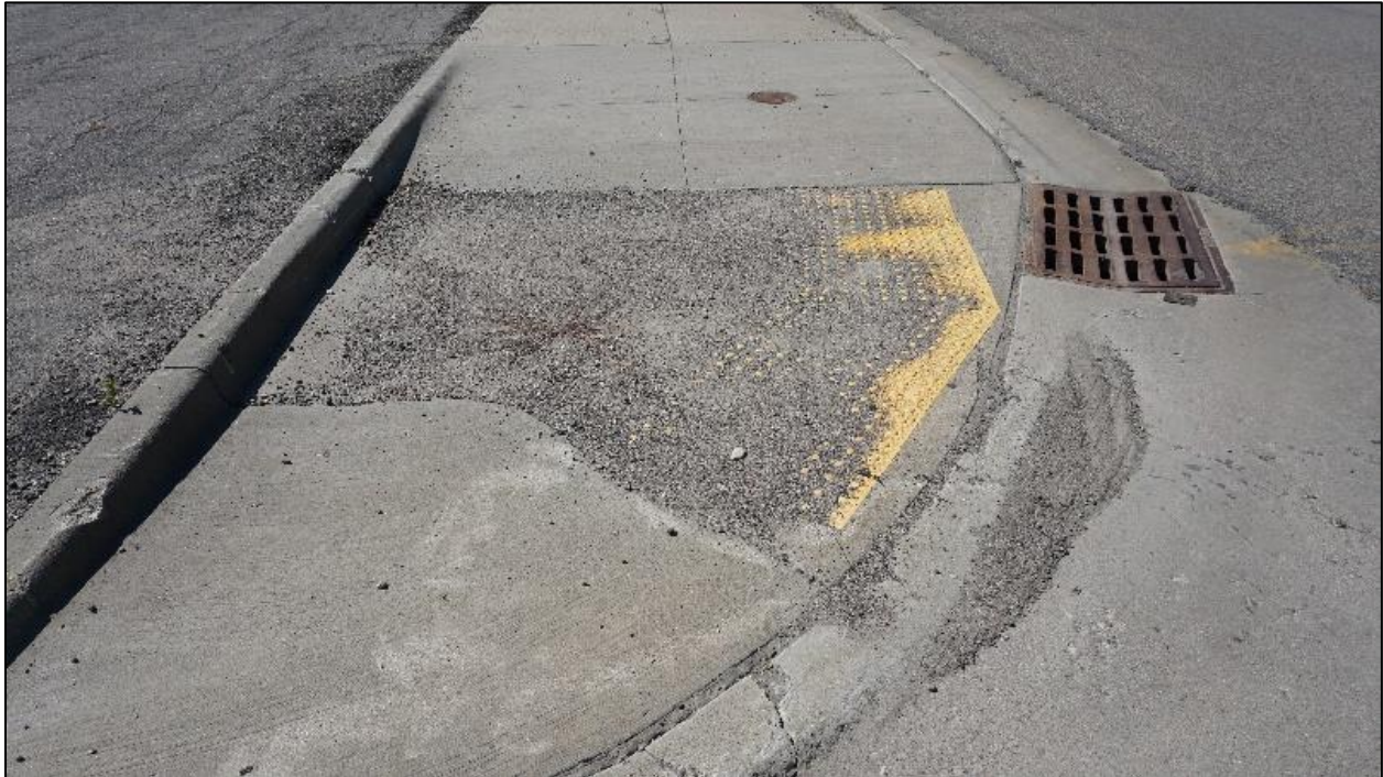
Figure 18. Debris strewn across ramp and potentially hazardous grate
