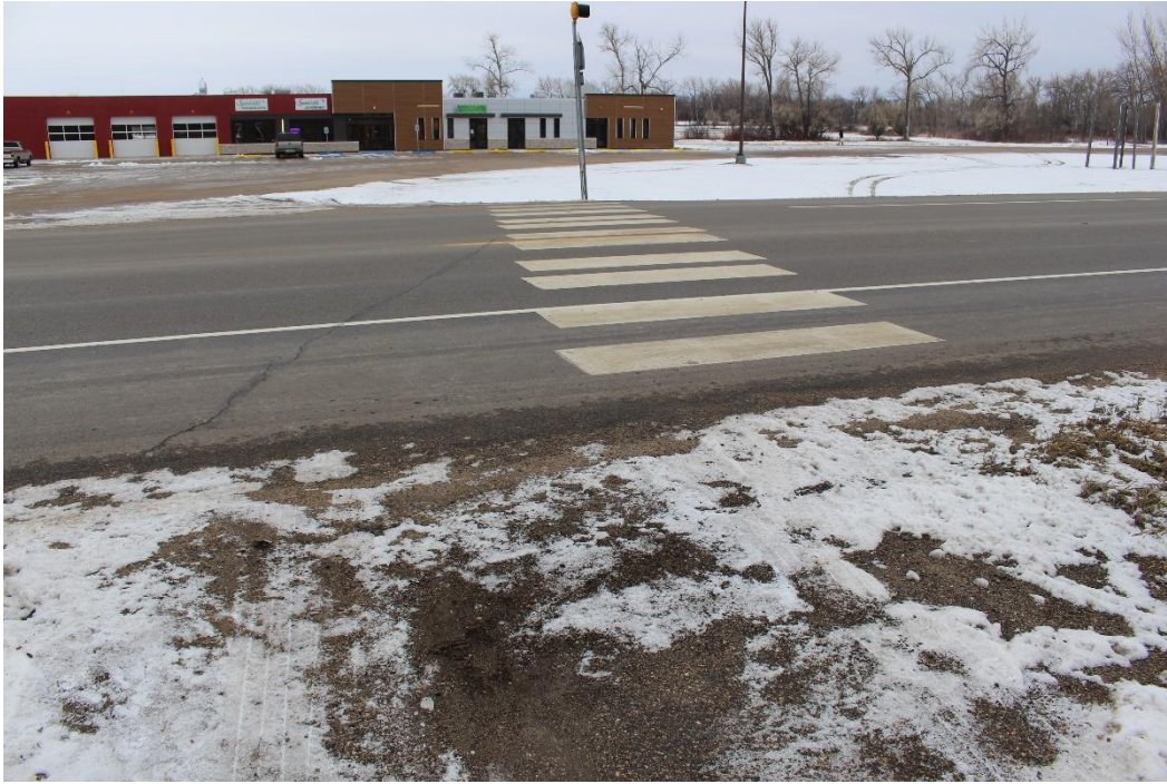
Figure 4. Missing ramp near Four Winds High School
