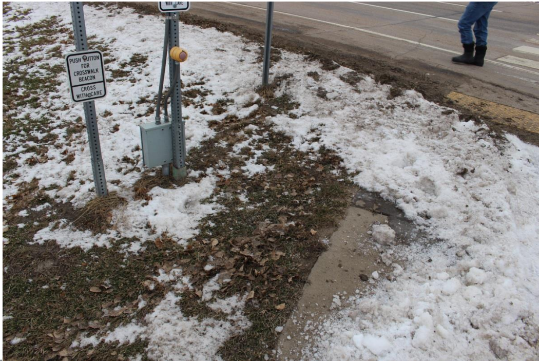
Figure 11. A location missing landing for the pedestrian push button
