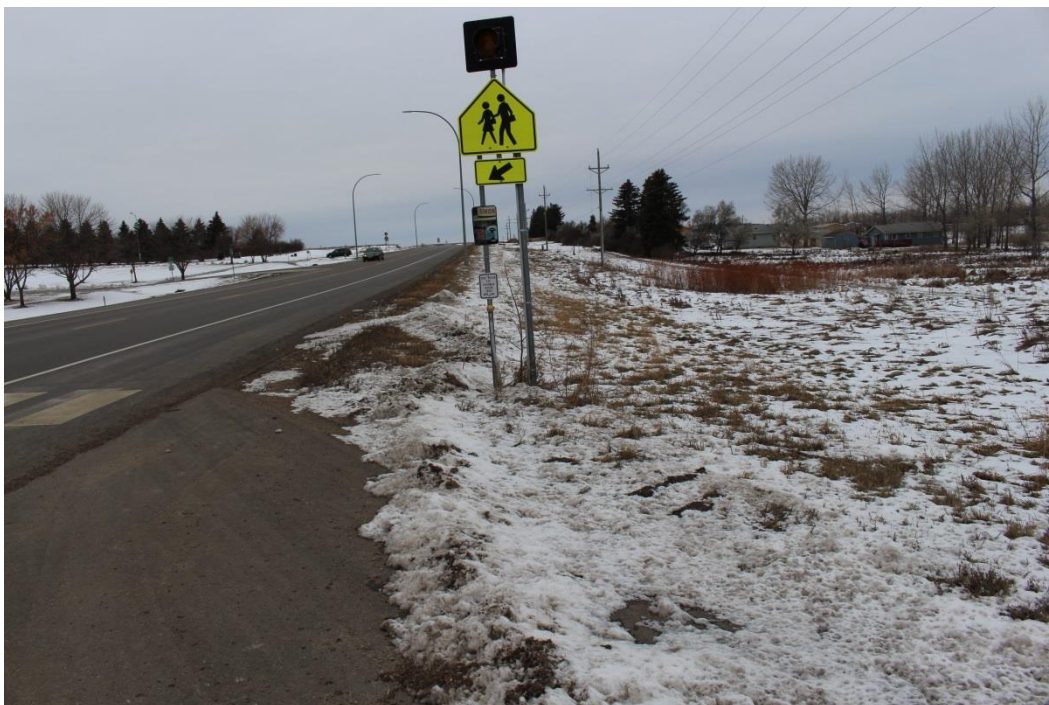
Figure 12. Another location with missing landing for pedestrian push button
