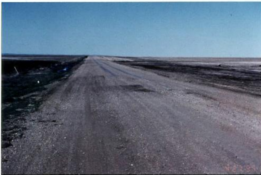
(Photographs of gravel-surfaced roadways in good condition)
