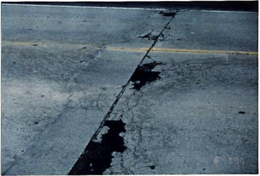
(Photographs of jointed concrete pavements in very poor or failed condition)
