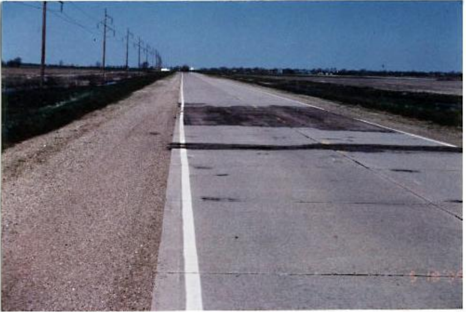
(Photographs of jointed concrete pavements in fair condition)
