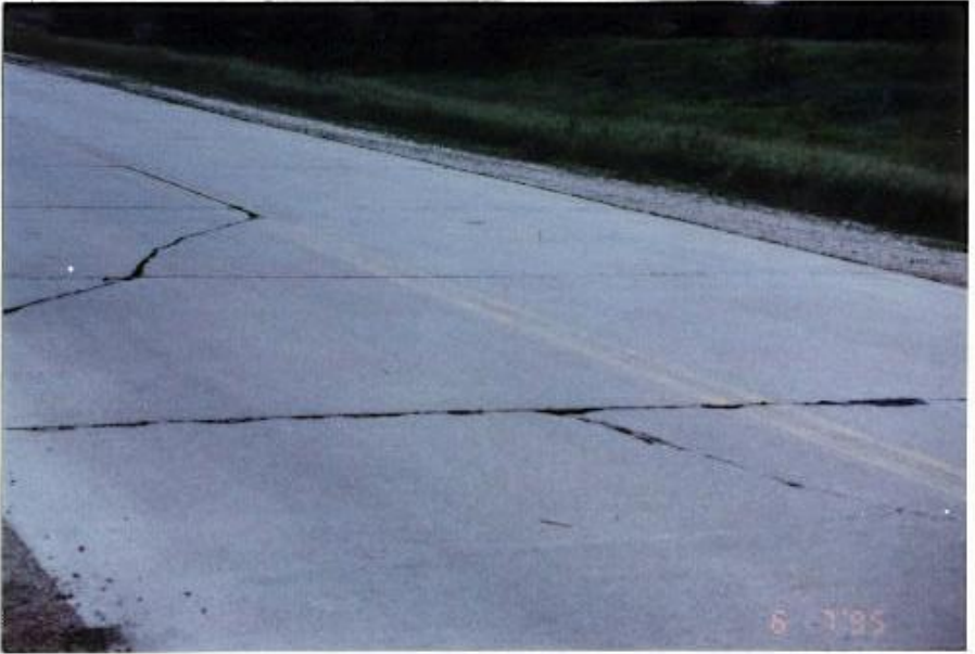
(Photographs of jointed concrete pavements in poor condition)
