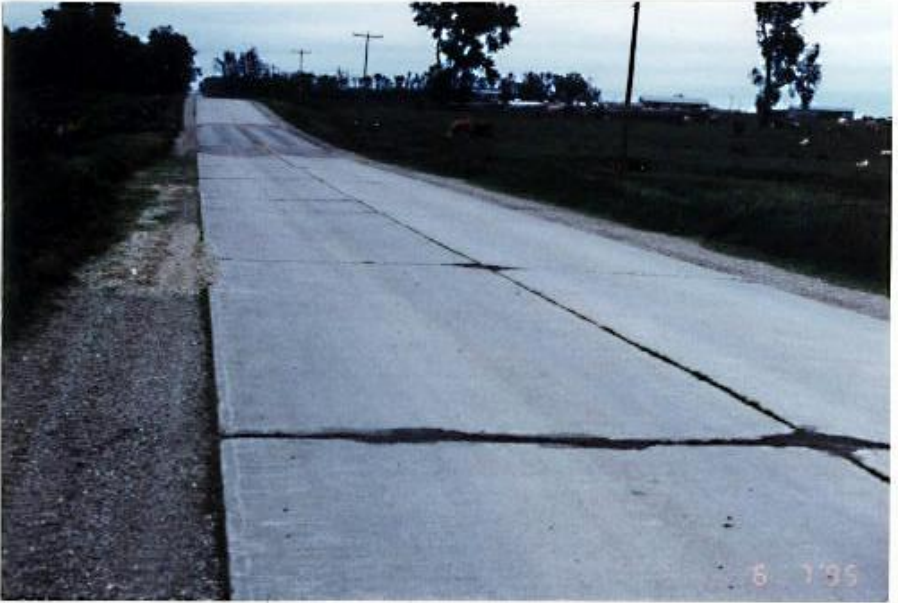
(Photographs of jointed concrete pavements in poor condition)
