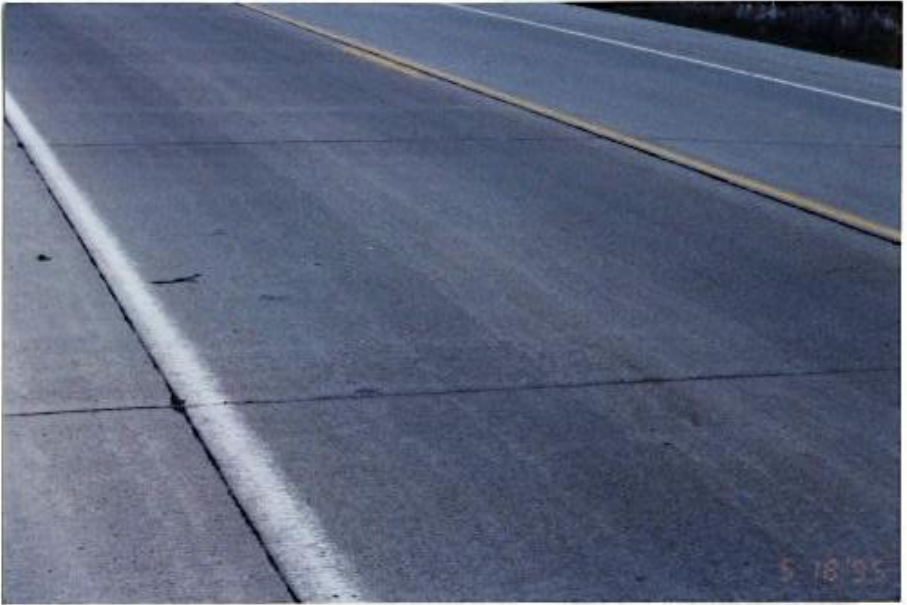
(Photographs of jointed concrete pavements in very good condition)
