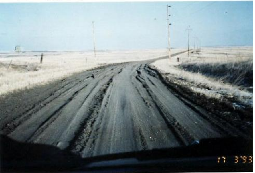
(Photographs of gravel-surfaced roadways in failed condition)
