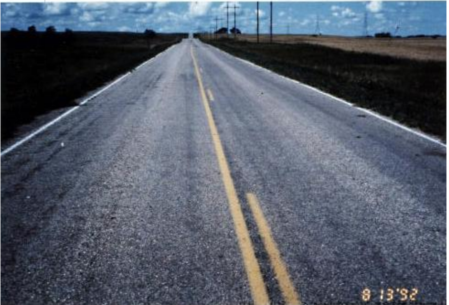
(Photographs of flexible pavements in very good condition)
