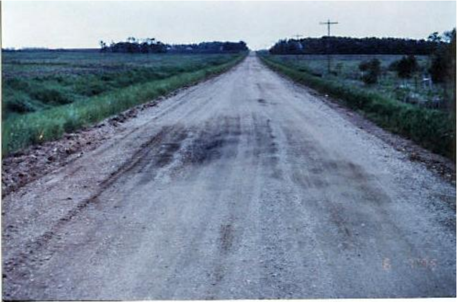
(Photographs of gravel-surfaced roadways in poor condition)
