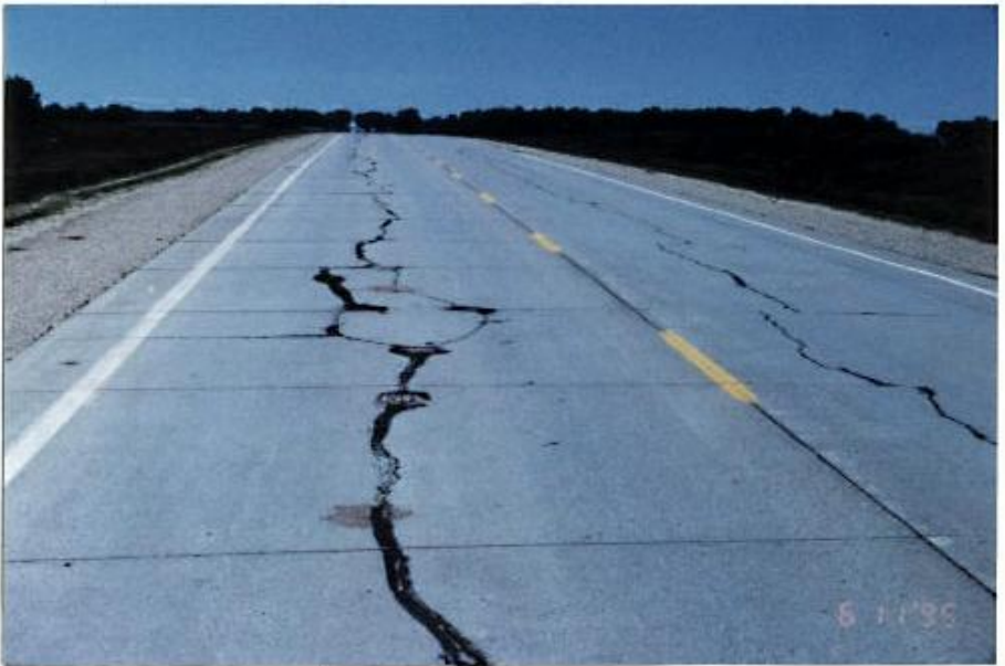
(Photographs of jointed concrete pavements in fair condition)
