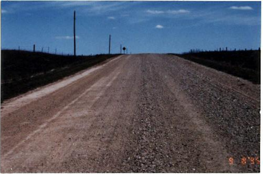
(Photographs of gravel-surfaced roadways in very good condition)
