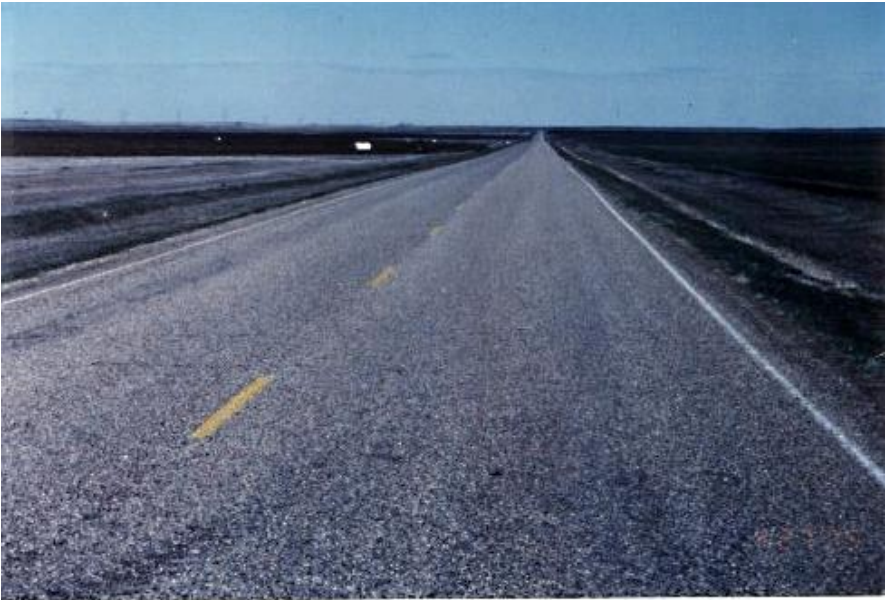
(Photographs of flexible pavements in very good condition)
