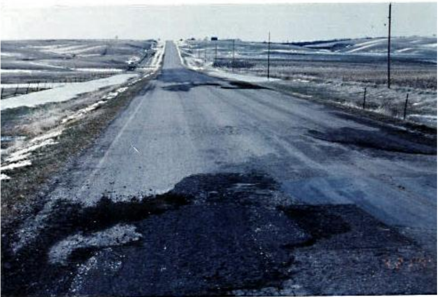
(Photographs of flexible pavements in poor condition)
