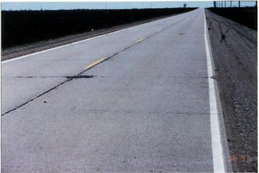
(Photographs of jointed concrete pavements in very good condition)
