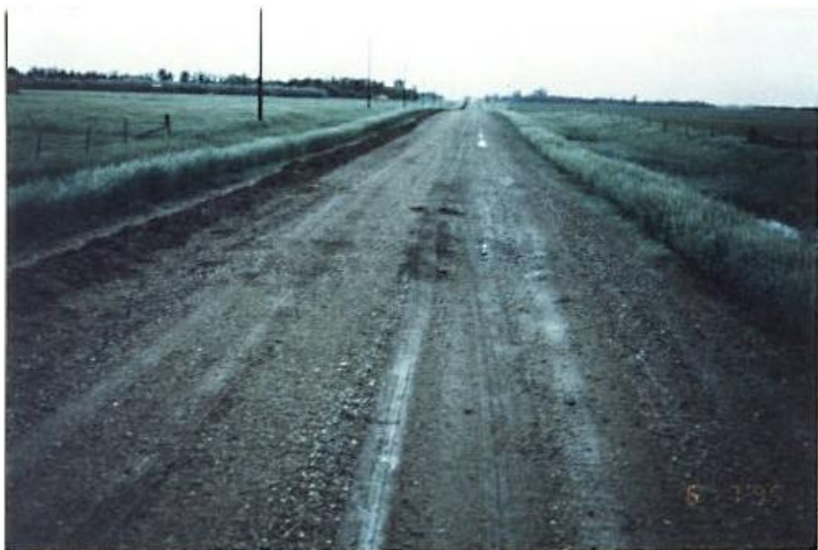
(Photographs of gravel-surfaced roadways in good condition)
