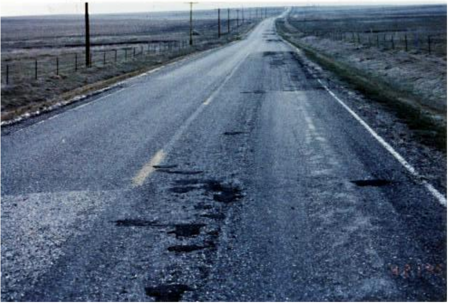
(Photographs of flexible pavements in fair condition)
