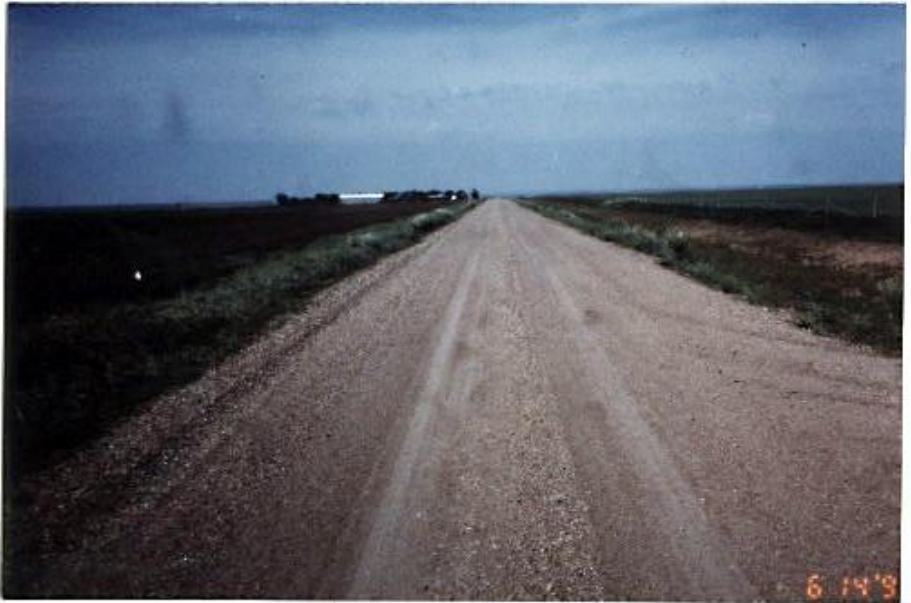
(Photographs of gravel-surfaced roadways in very good condition)
