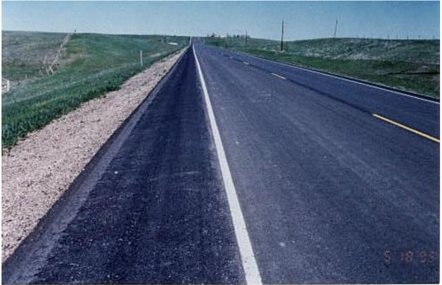
(Photographs of flexible pavements in excellent condition)
