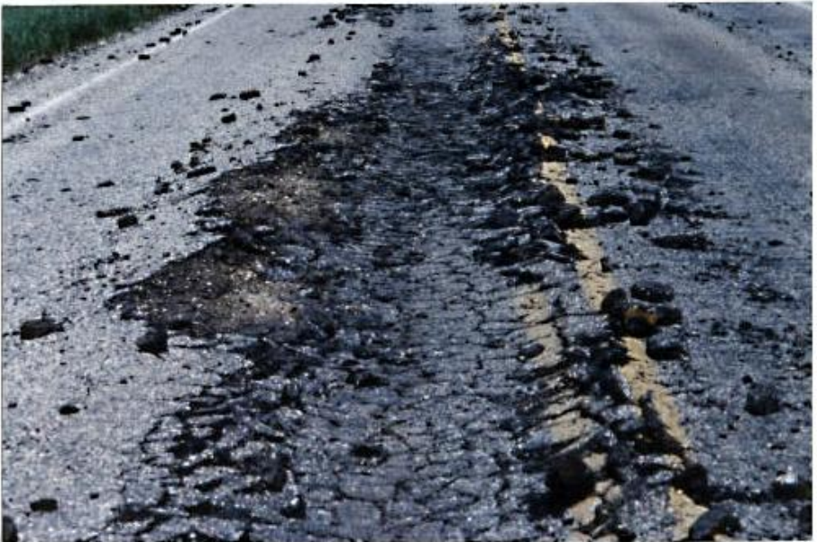
(Photographs of flexible pavements in very poor to failed condition)
