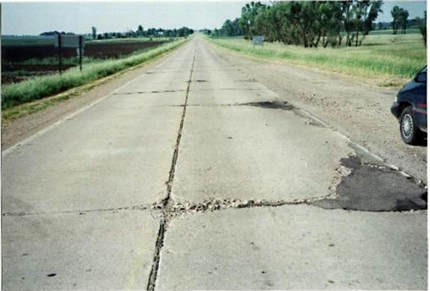
(Photographs of jointed concrete pavements in very poor or failed condition)
