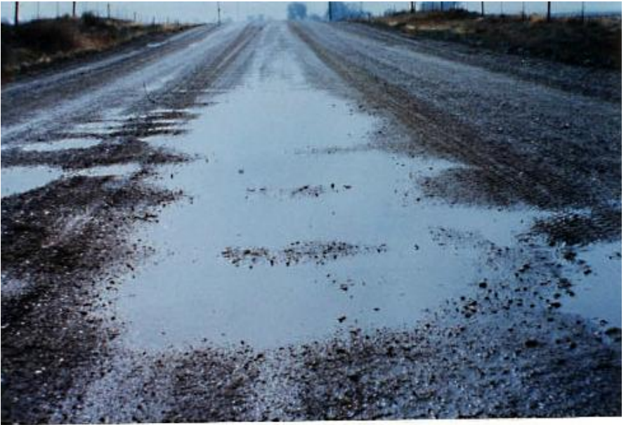
(Photographs of gravel-surfaced roadways in failed condition)
