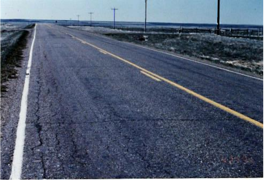
(Photographs of flexible pavements in fair condition)
