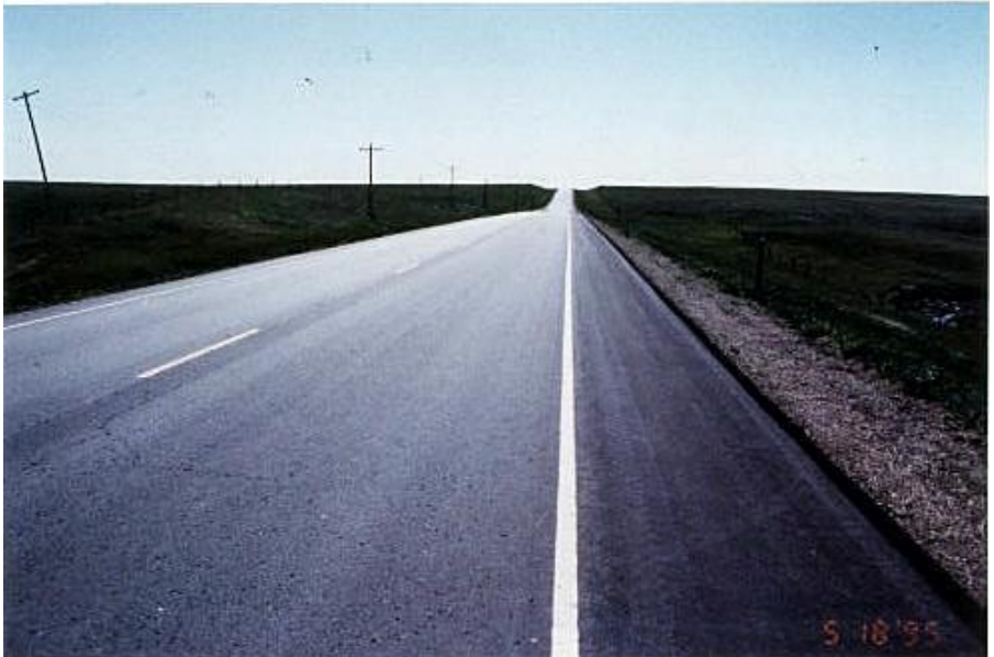
(Photographs of flexible pavements in excellent condition)
