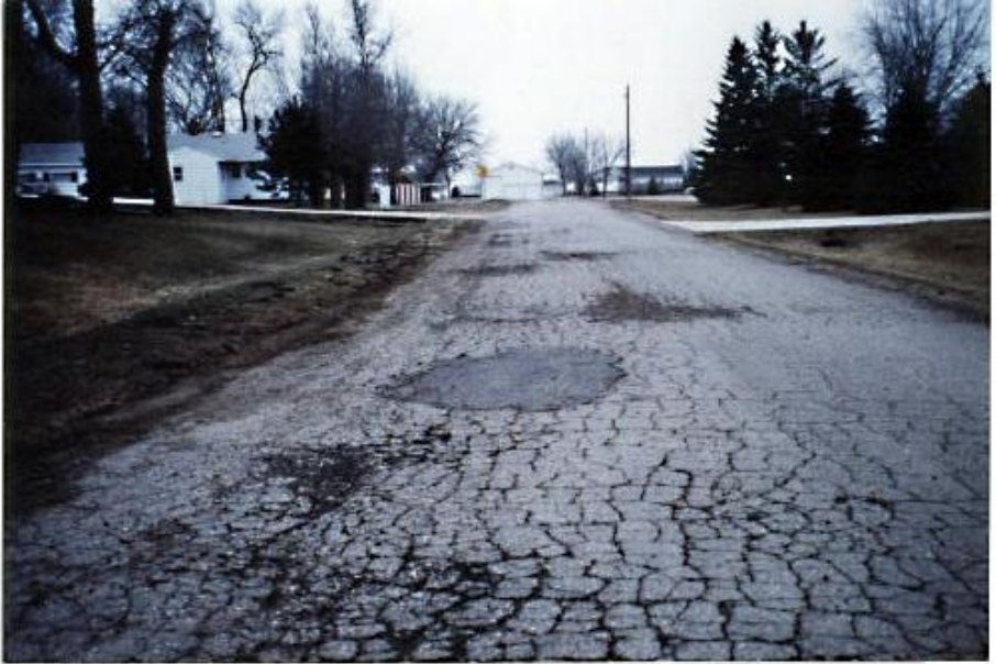
(Photographs of flexible pavements in very poor to failed condition)
