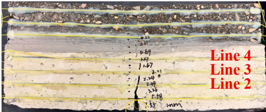
Figure 9. Post-test fracture pattern of the rectangular asphalt-overlaid PCC specimen following three-point bending
