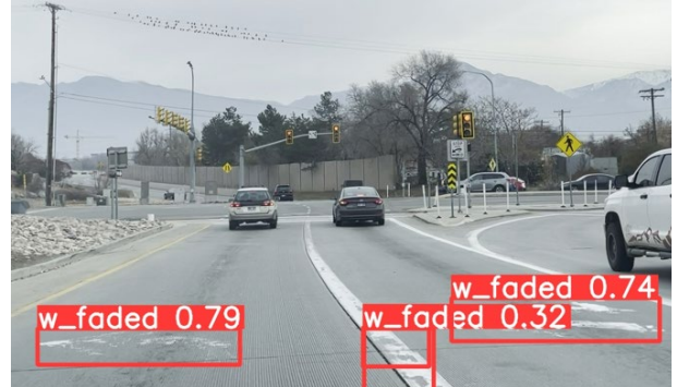
(f) Faded White Arrow and Lane Markings-2
