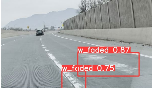
(e) Faded White Arrow and Lane Markings-1
