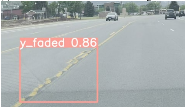
(g) Faded Yellow Single Lane Marking
