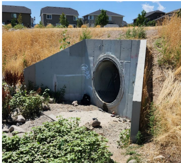
Figure 1. Culvert under a road
