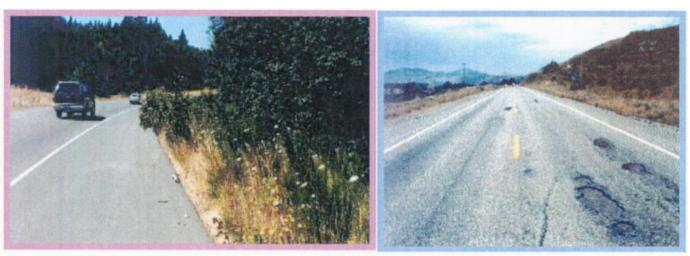
nificantly obscuring ditch lines, guardrail, of striping, signage, and delineators have lost night reflectivity, are worn or missing. Guardrail has sustained significant visible damage and moderate structural deterioration. Storm drains have significant blockages. Erosion or slides may encroach or threaten the roadway. Standing water visible in the travel lane(s) during a normal storm event.
