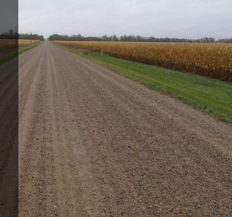
Substandard section – aggregate has moved outward nearly 4 ft since construction
