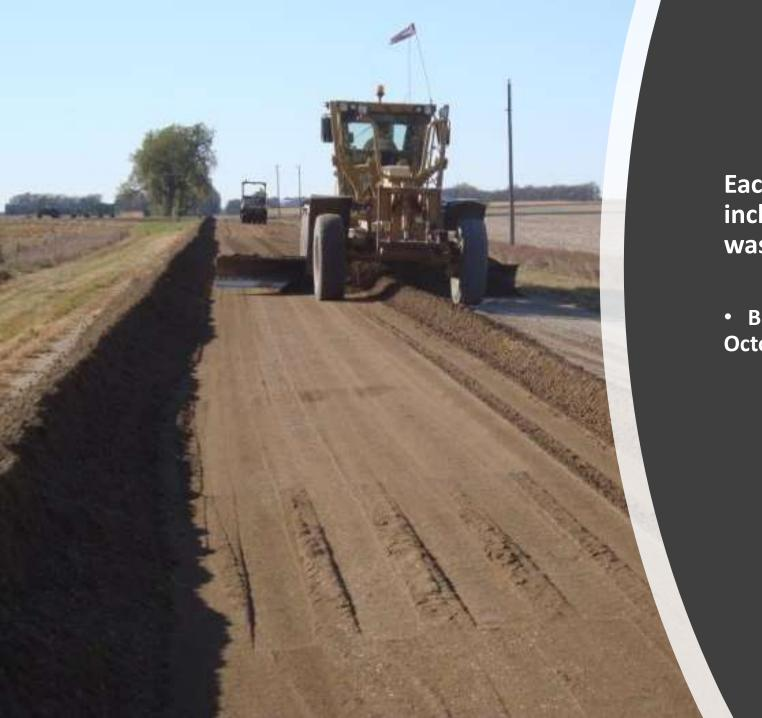
Each section was built with three to four inches of new gravel after existing surface was prepared and shaped.
