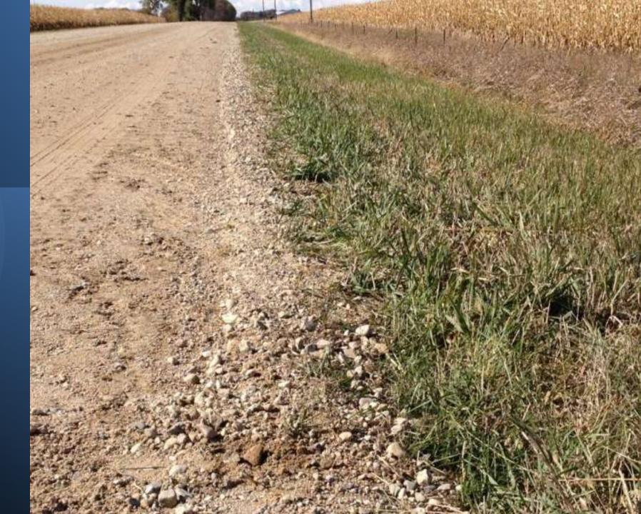
Modified section has moved outward only six inches since construction
