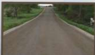
1/4 GOOD: 6-6-13 Just after treatment at 0.5 gal per sq yd. Commercial dairy road. Heavy truck traffic -AADTT 30 - 40. Road looks good.
