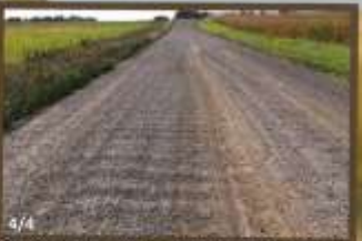
4/4 POOR: 10-7-13 After another 0.3 gal per sq yd was applied same season still not performing well. This is such poor surface material it won't go into a bound state no matter how you maintain it. There is no way the MgCl_2 can work even with 0.8 gal per sq yd applied in one year!
