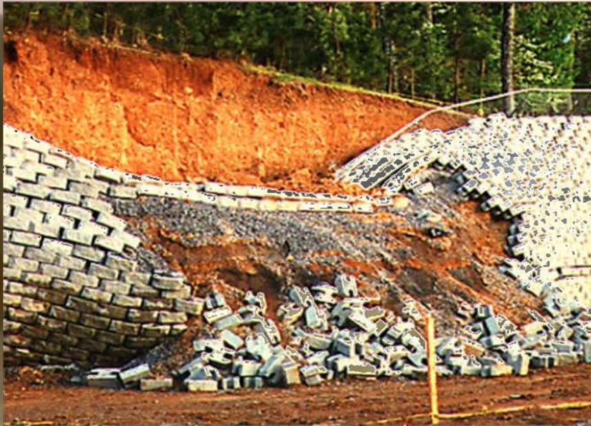
No reinforcement
