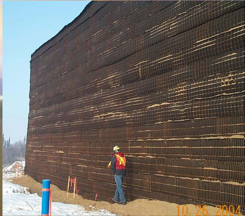
Welded Wire Basket Bridge Abutment
