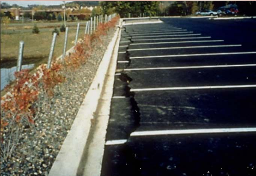
Poor Compaction
