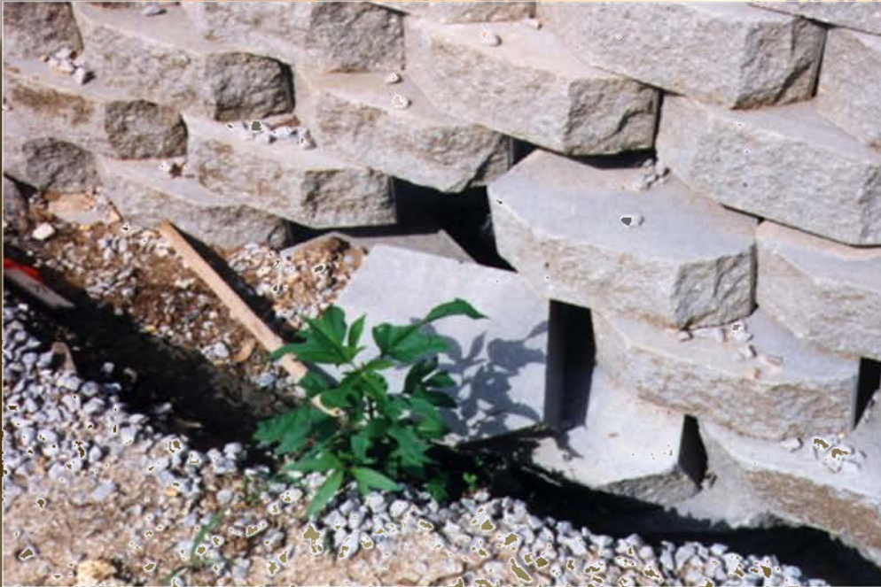
Incorrect drainage
