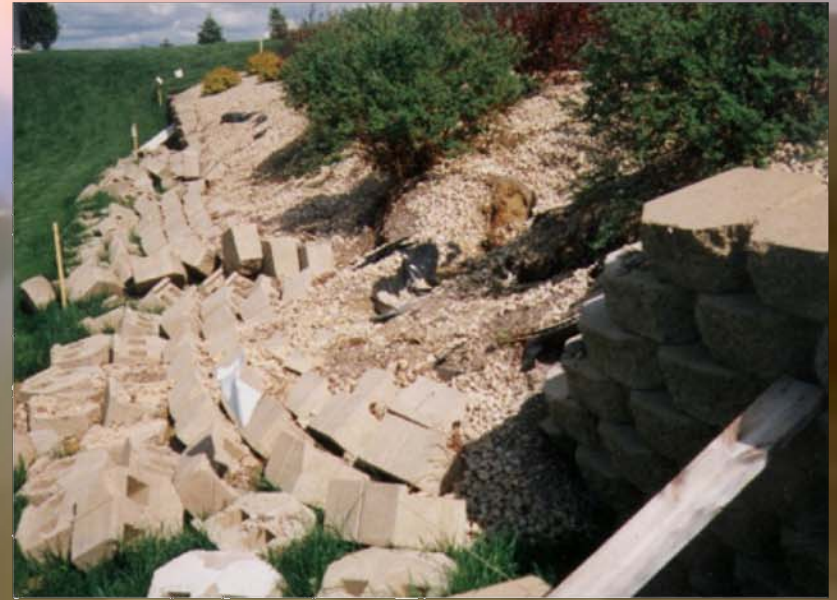
Incorrect reinforcement
