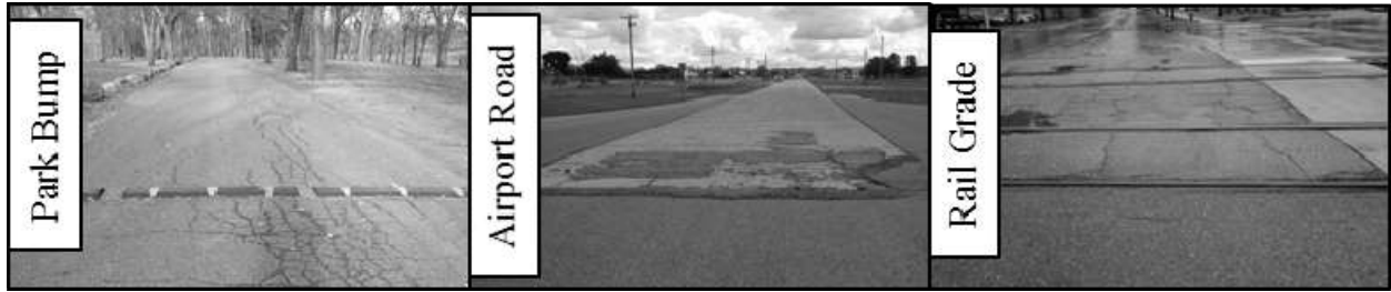
Figure 1. Isolated anomalies traversed for the case study measurements.
