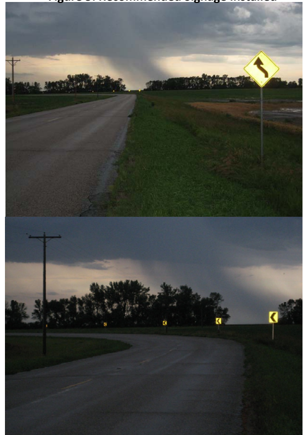
Figure 5: Recommended Signage Installed
