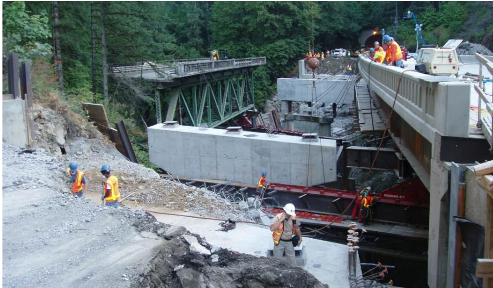
Lateral Bridge Slide in Oregon “ABC—Experience in Design, Fabrication, and Erection of PBES”
