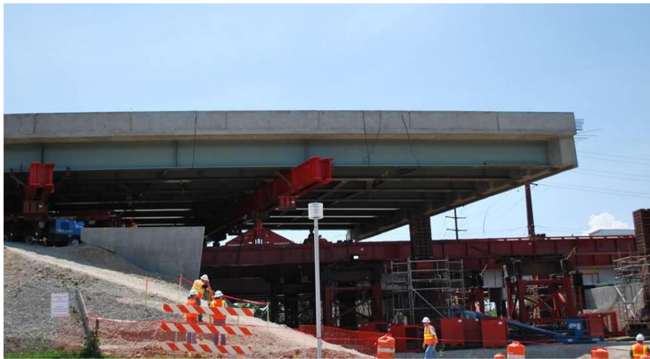
Longitudinal Launching of a Utah Bridge “ABC—Experience in Design, Fabrication, and Erection of PBES”
