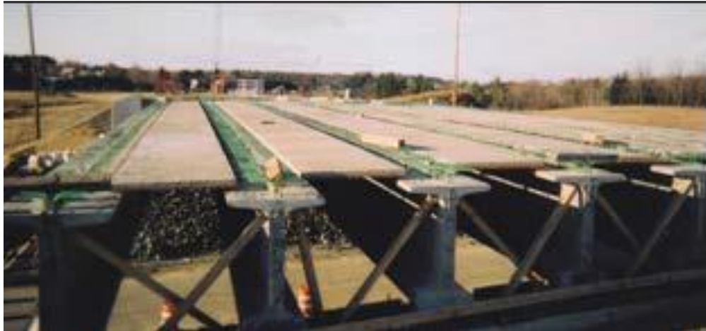
Partial-Depth Precast Deck Panels http://www.fhwa.dot.gov/bridge/abc/prefab_def.cfm Accessed 23 Oct 2012
