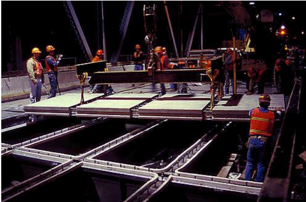
Steel Grid System with Full-Depth Precast Concrete Deck Installation “ABC—Experience in Design, Fabrication, and Erection of PBES”
