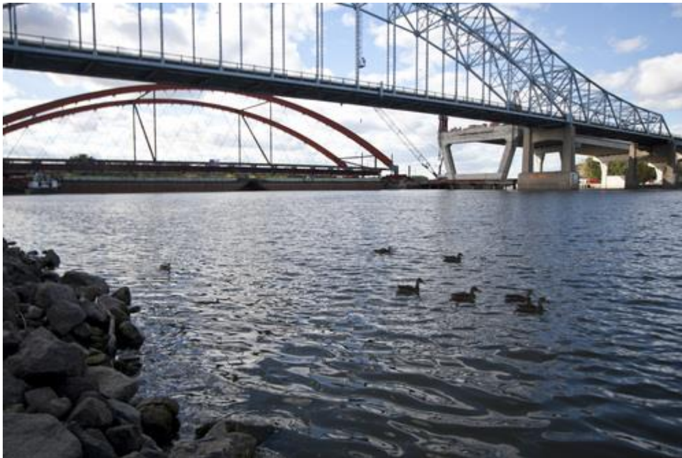
Hastings, MN Tied Arch Bridge on Barge Before Being Lifted into Place http://www.hastingsstargazette.com/event/photogallery/id/57/ Accessed 23 Oct 2012
