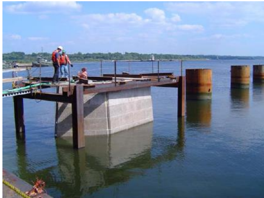
Example of a Precast Pier Box Cofferdam http://www.fhwa.dot.gov/bridge/prefab/if09010/04.cfm Accessed 23 Oct 2012
