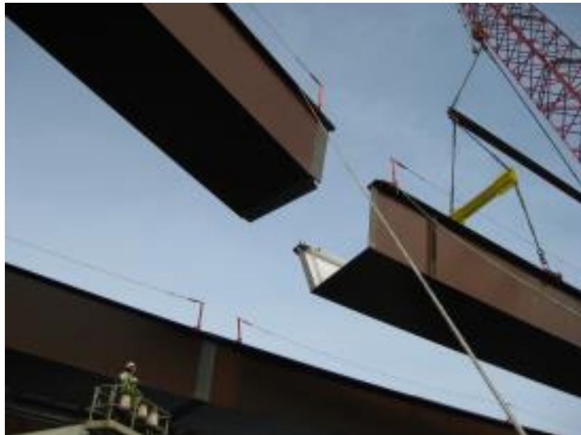
Steel Tub Girder Placement
