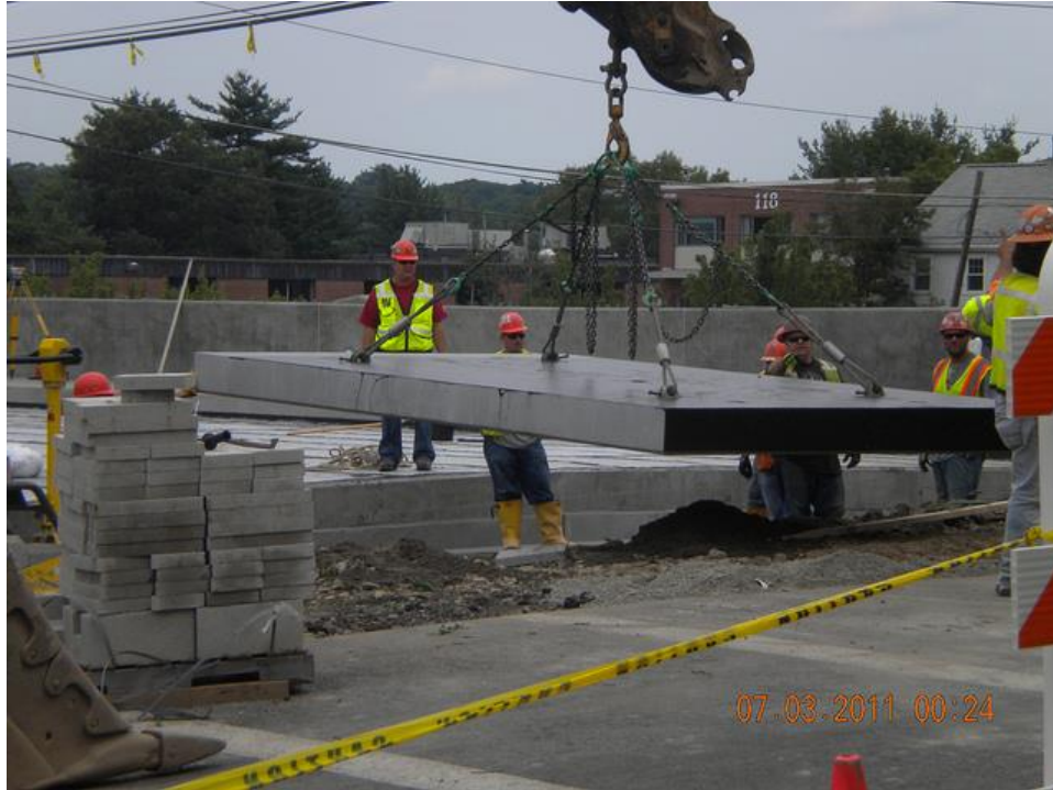
Precast Approach Slab Installation http://www.flickr.com/photos/25664139@N06/5899098381/ Accessed 16 Nov 2012
