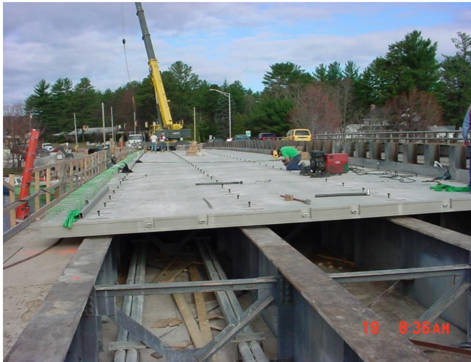
Full-Depth Precast Deck Panels “ABC—Experience in Design, Fabrication, and Erection of PBES”
