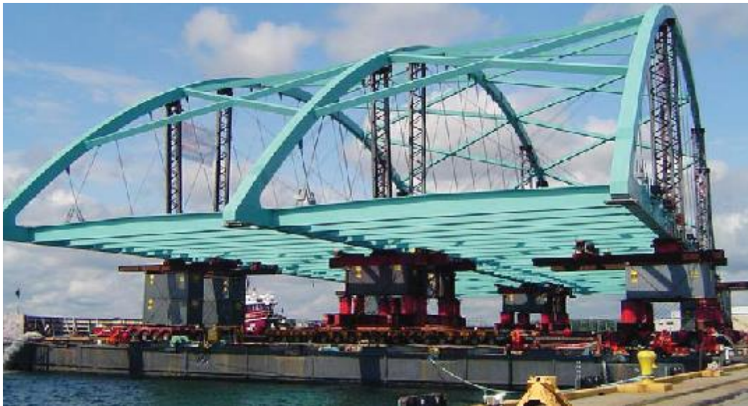
Replacement of Truss Span without Deck (Barge Use) http://www.fhwa.dot.gov/bridge/abc/docs/aashto.pdf Accessed 23 Oct 2012
