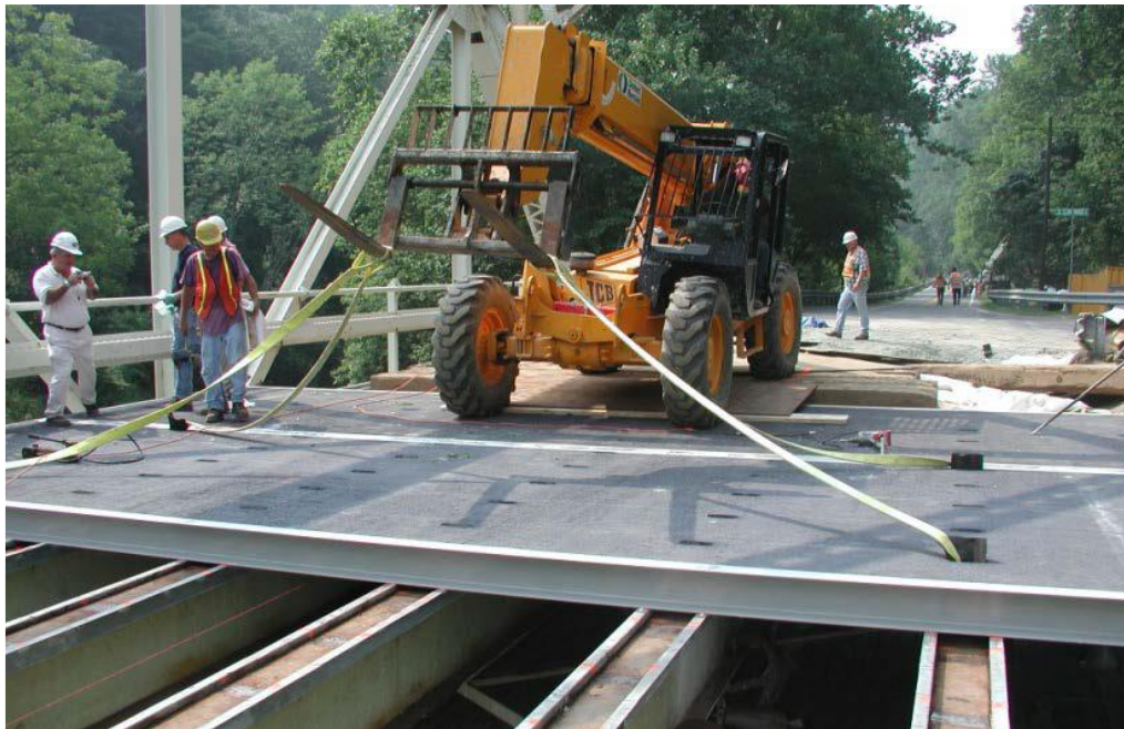
Full-Depth FRP Panels “ABC—Experience in Design, Fabrication, and Erection of PBES”
