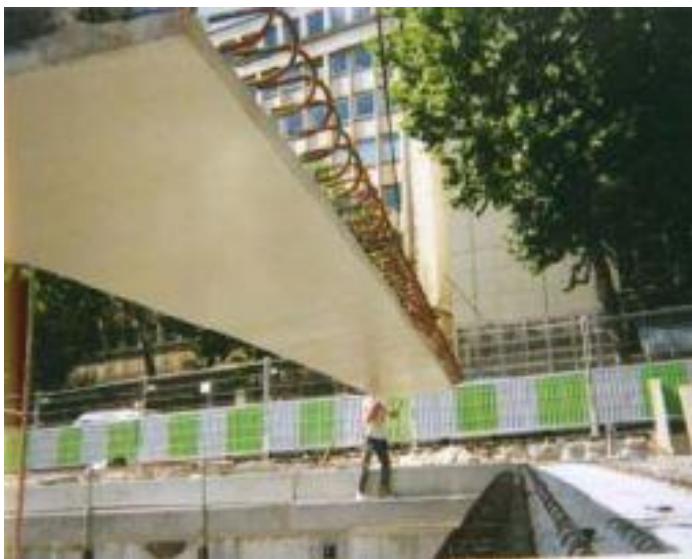
Inverted T Bridge System http://www.fhwa.dot.gov/bridge/prefab/slab.cfm Accessed 15 Nov 2012
