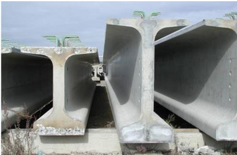
Precast Bulb-T Girders
