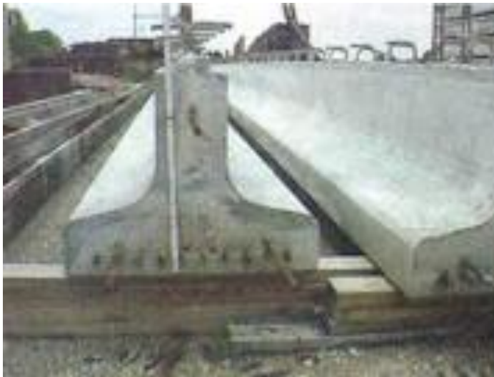
Precast Inverted T-Beam http://rebar.ecn.purdue.edu/ect/links/technologies/civil/itbeam.aspx Accessed 23 Oct 2012
