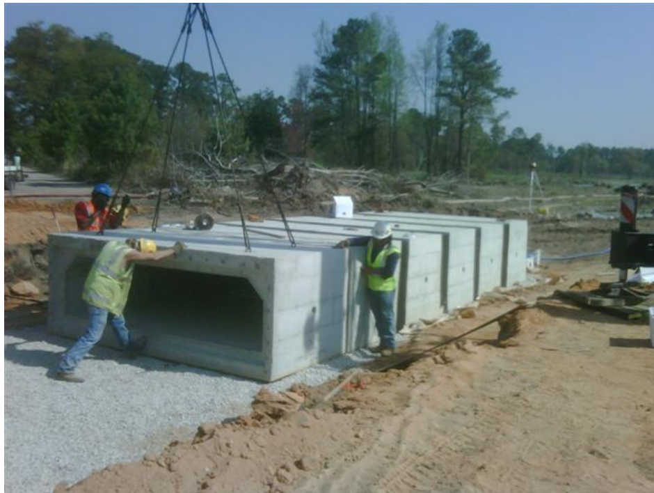
Precast Box Culvert Assembly http://www.mcprecast.com/products.asp Accessed 16 Nov 2012
