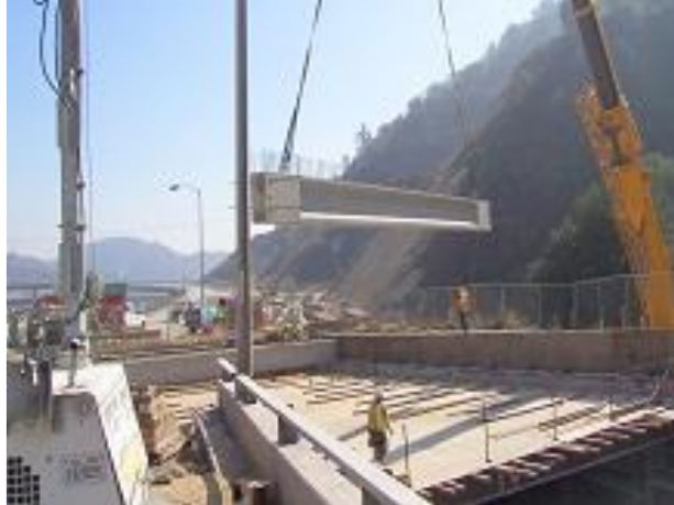
Placement of a Precast I-Girder at the Job Site “ABC Applications in CA—A Lesson Learned”
