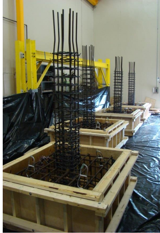
(b) Completed Footing/Column Steel Cage
