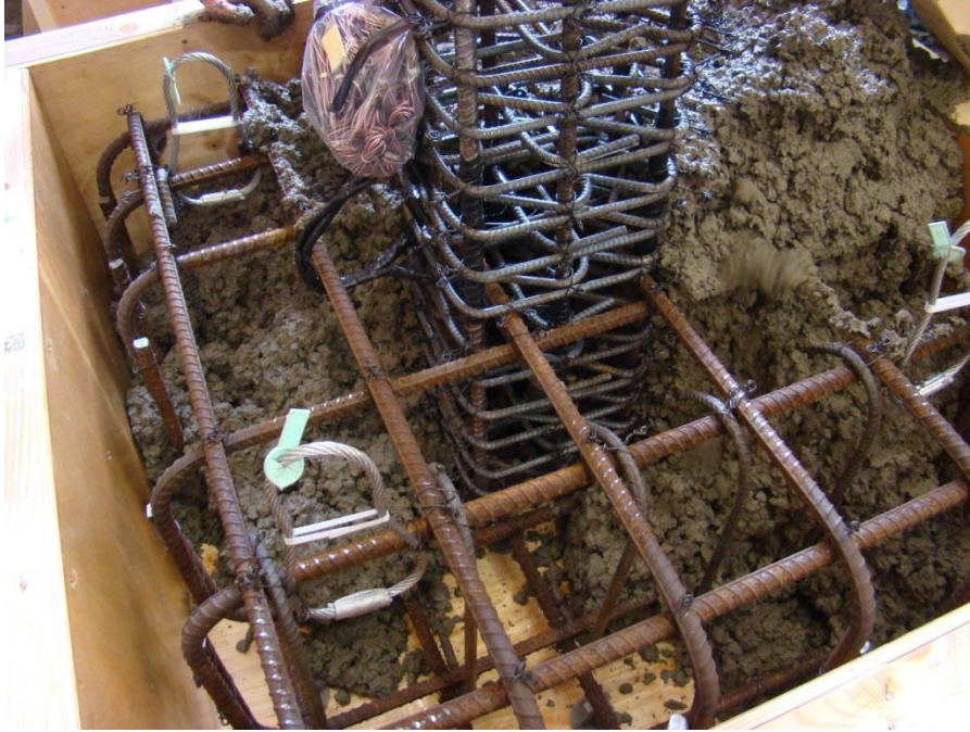
Figure 1.1 Placement of Conventional Concrete in a Highly Congested Bridge Column-Footing Connection
