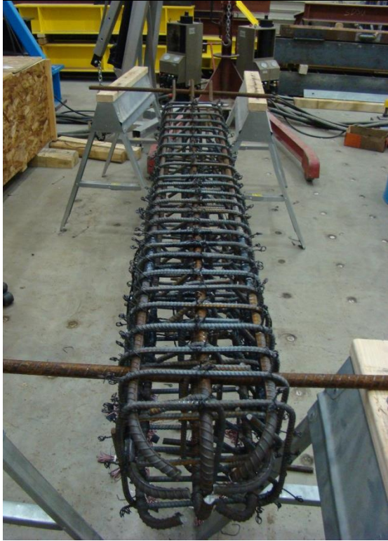
(a) Column Steel Cage
