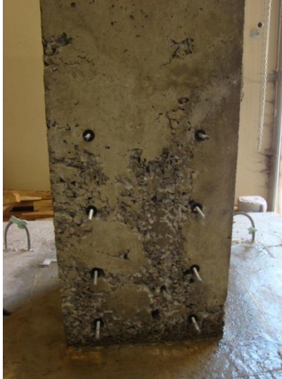
Figure 4.24 Specimen SCC2 Plastic Hinge Region Concrete Defects (Looking North)
