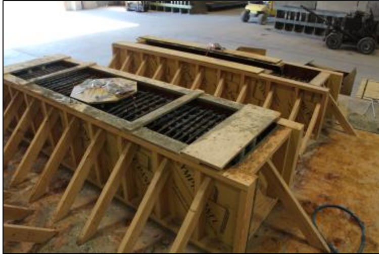
Figure 2.29 FGSS-2 precast components inside concrete forms.
