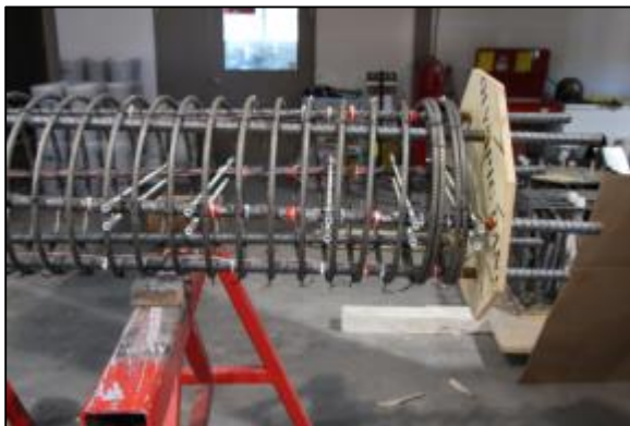
(a) Column cage with projecting bars.
