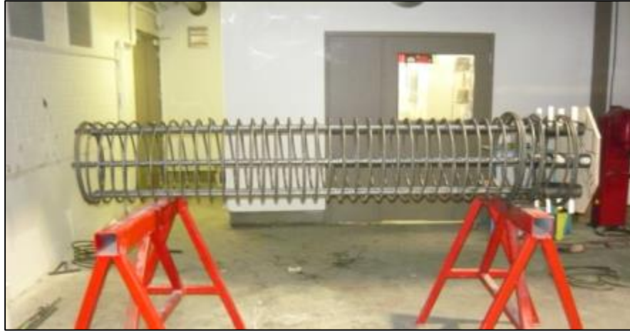
(a) Column rebar cage.
