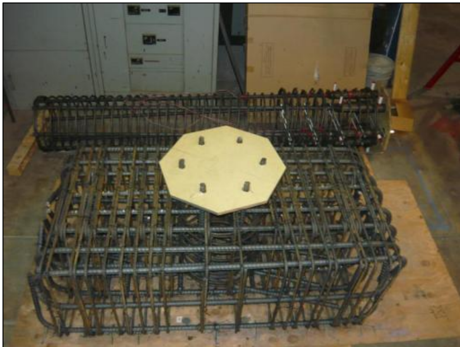
(b) Column and footing rebar cages.
