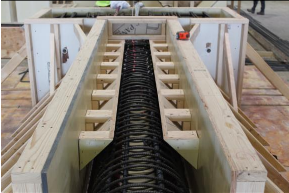
Figure 2.18 GGSS-CIP rebar cage inside form.
