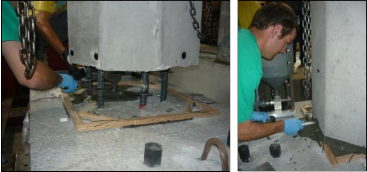
Figure 2.7 Grouting operation for GGSS-1.
