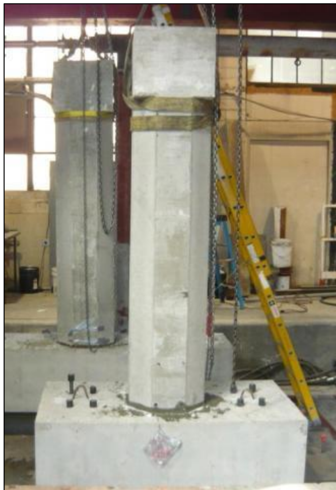
Figure 2.8 GGSS-1 in the final position.
