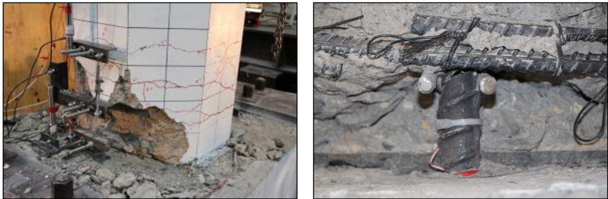
(b) Damage state at 7% drift ratio: cracks, spalling, fractured bar, and exposed rebar cage.
