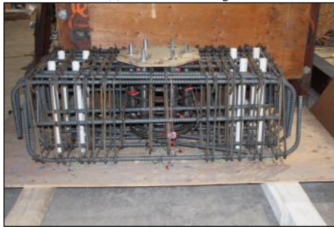
(b) Footing rebar cage.
