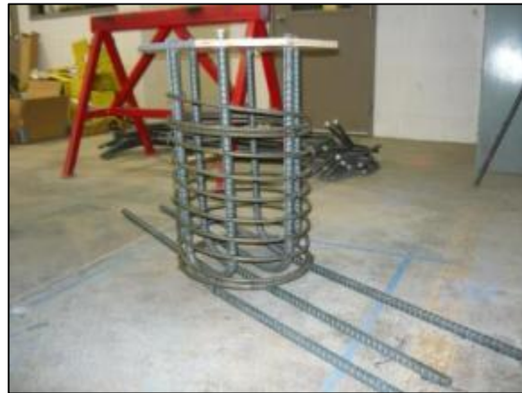
(b) Footing dowel bars with inward tails.
