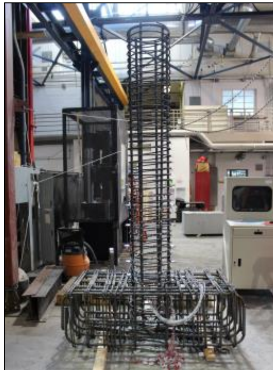
(b) Rebar cage ready to cast concrete.
