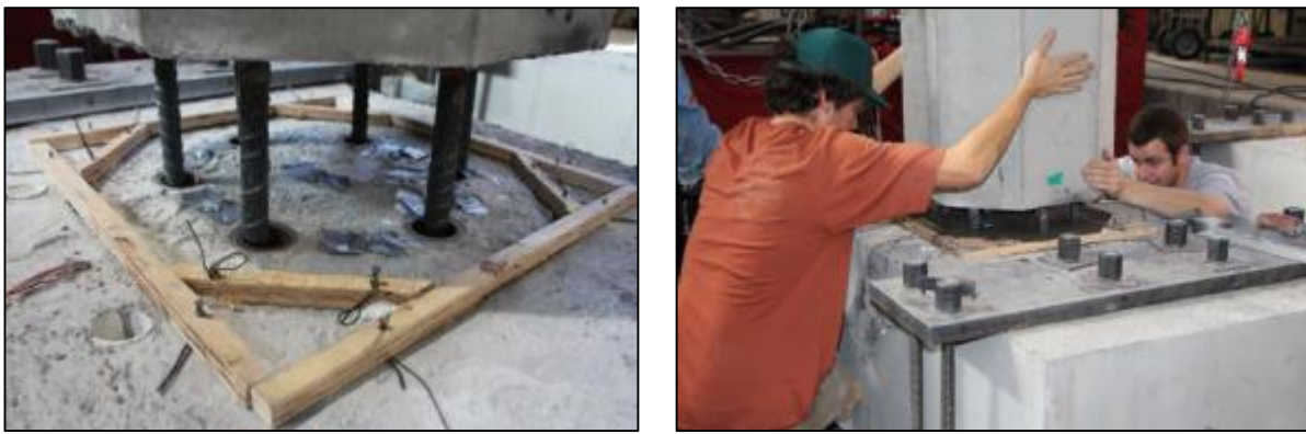
Figure 2.14 Grouting operation for GGSS-2.
