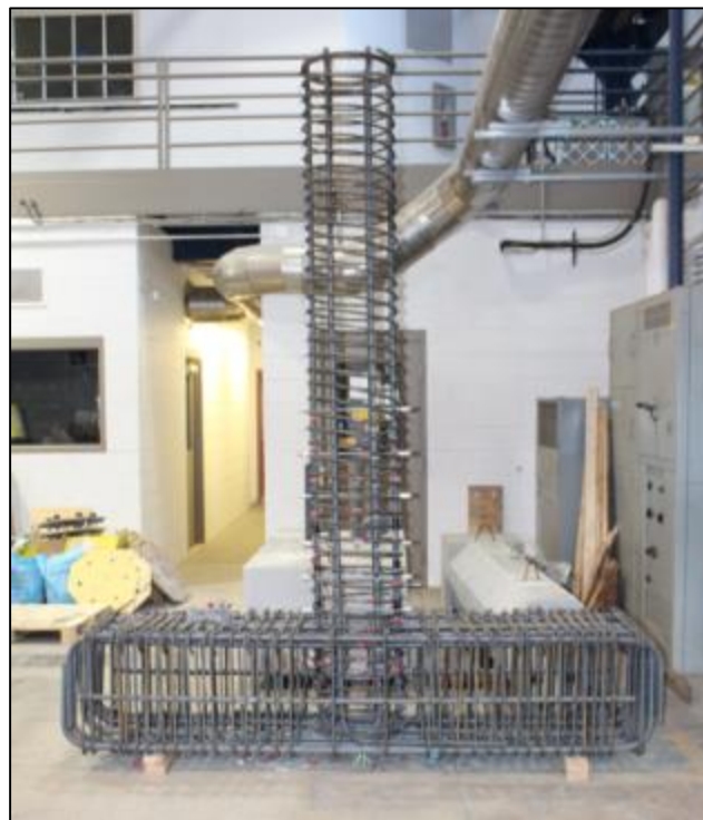
(b) Rebar cage ready to cast concrete.
