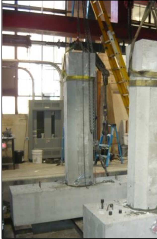
Figure 2.25 FGSS-1 (back) in final position.
