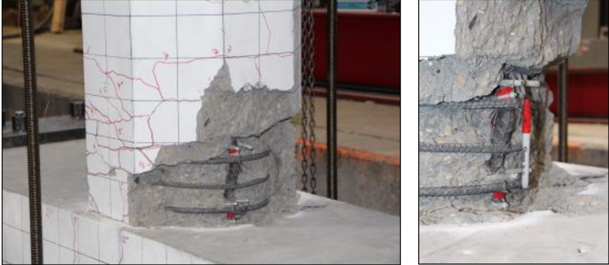
Figure 4.41 Damage state for FGSS-CIP: cracks and spalling, rebar buckling and fracture.
