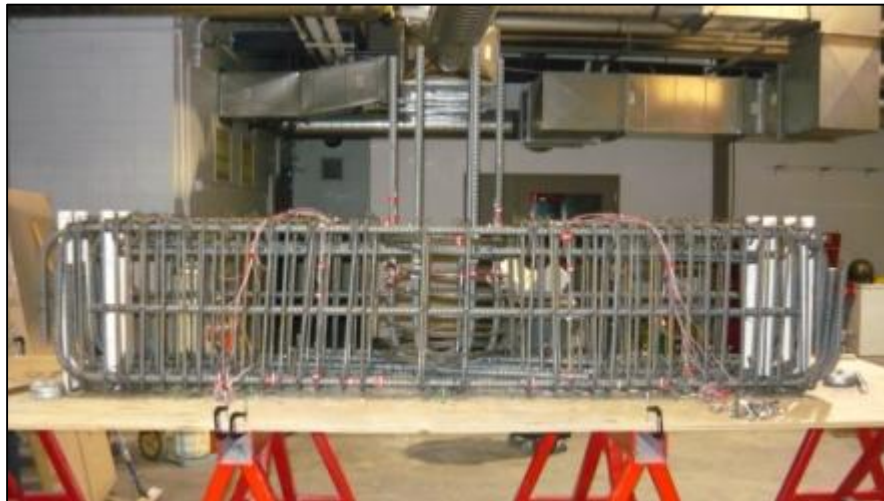
(c) Cap beam rebar cage.
