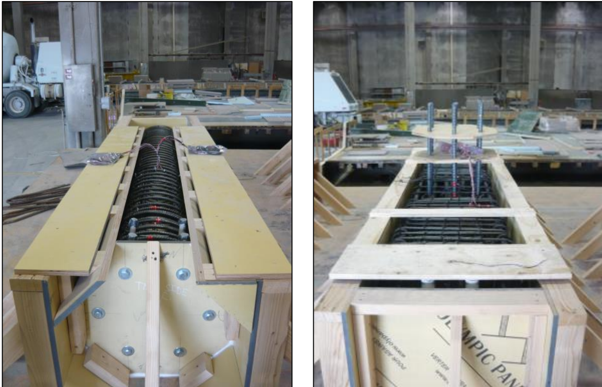
Figure 2.23 FGSS-1 precast components inside concrete forms.
