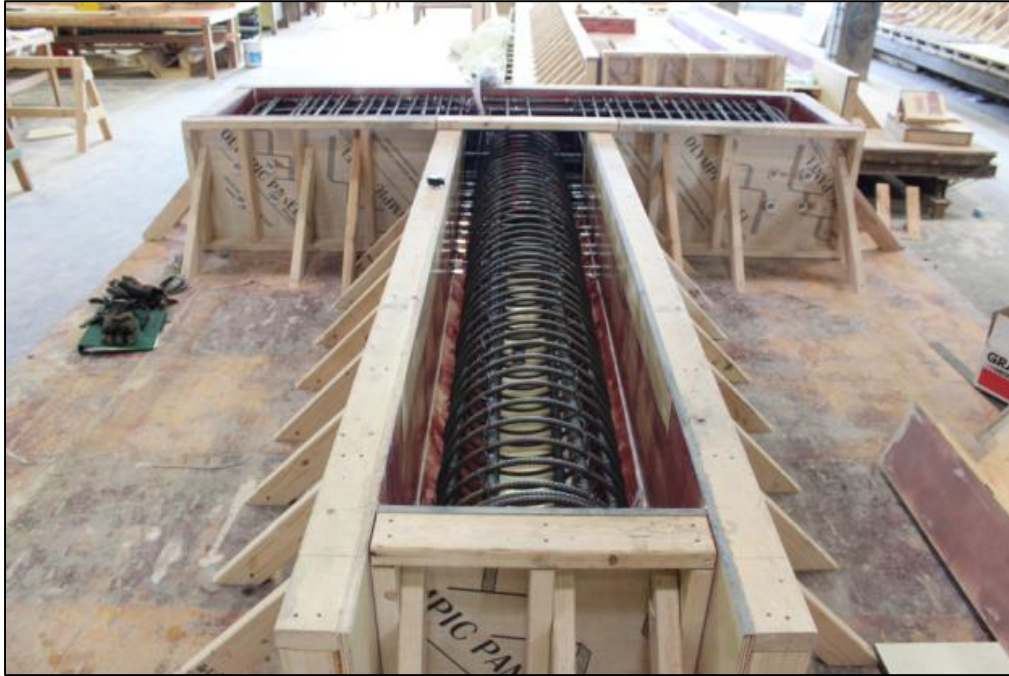
Figure 2.34 FGSS-CIP rebar cage inside form.
