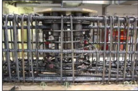
(b) FGSS placed within cap beam.
