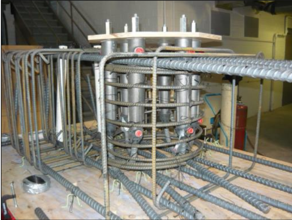
Figure 2.10 GGSS-2 precast footing core rebar cage.
