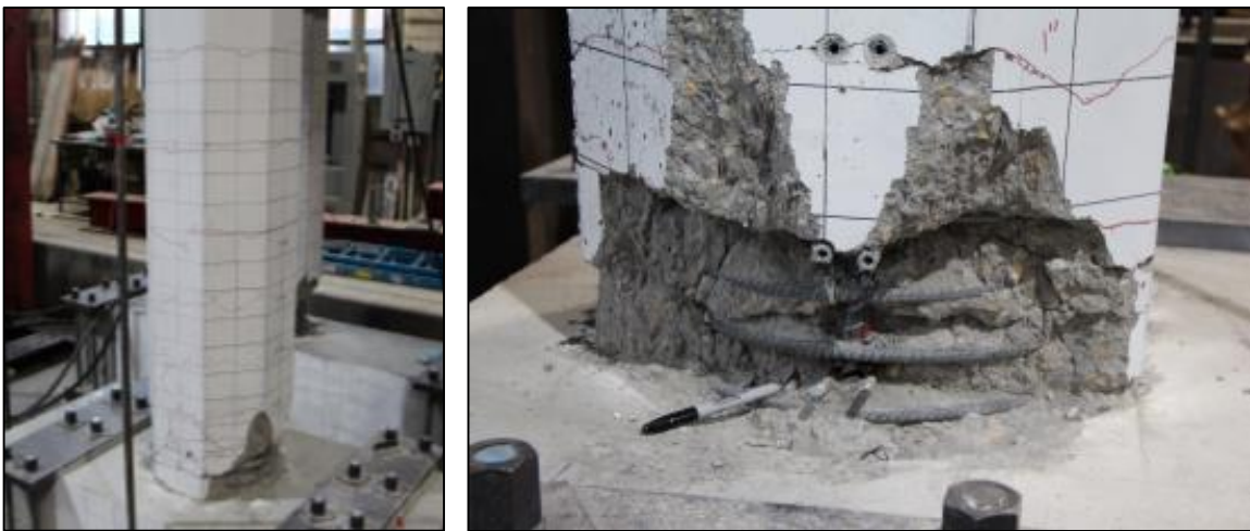
(c) Damage state at end of test: cracks, spalling, concrete delamination, and fractured rebar.
