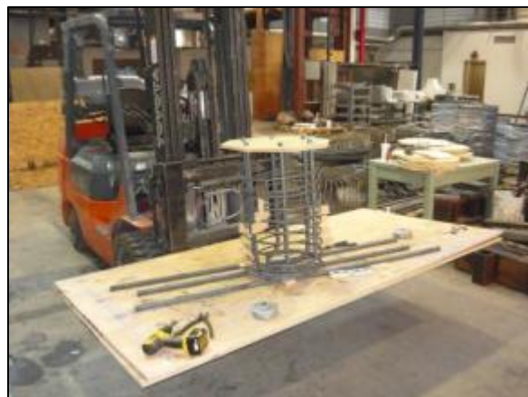
(b) Cap beam dowel bars with inward tails.
