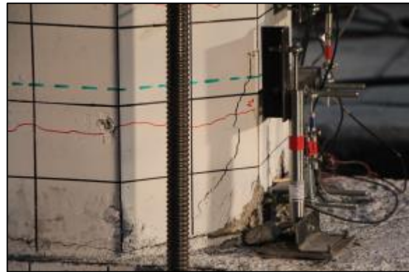
(b) Damage state at 3% drift ratio.
