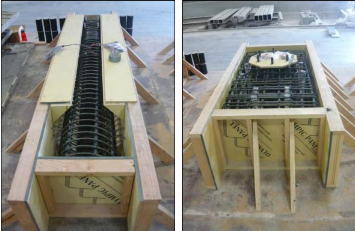
Figure 2.6 GGSS-1 precast components inside forms.
