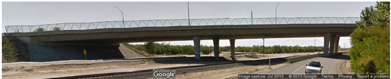
Figure C.2 Picture of on-site bridge (Image capture July 2012, Map data ©2015 Google)
