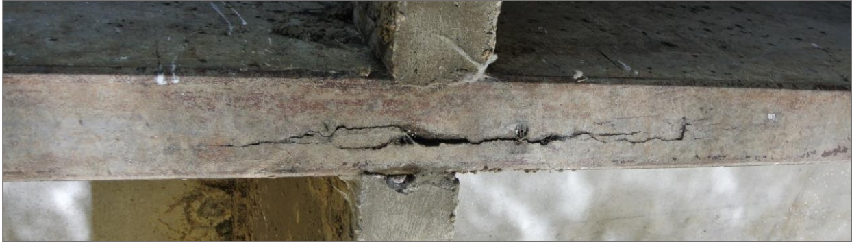
Figure 8.6 Longitudinal crack on Girder B at midspan
