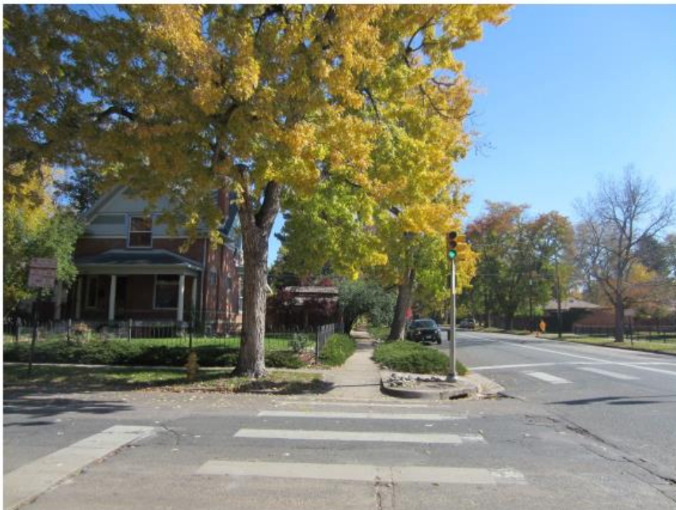
Crosswalks were marked and sidewalks were well maintained with curb ramps on all four corners of the intersection of 23rd and Dexter.
