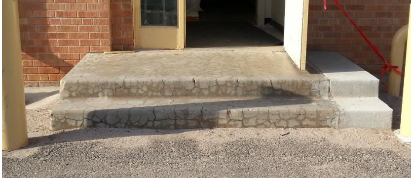
Figure 3.2 Wyoming steps used as aggregate for RCA-S study.
