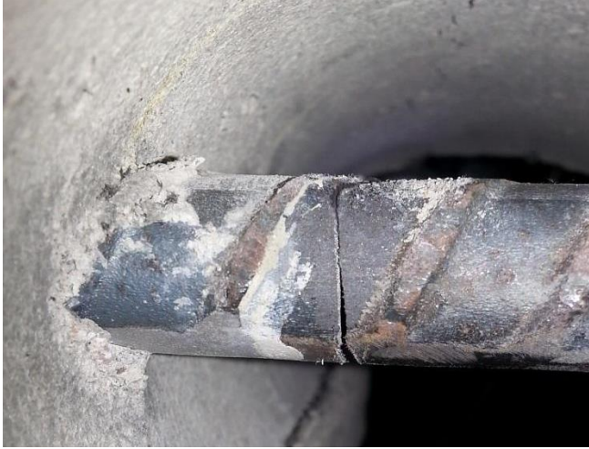
Figure 4.4 Fatigue induced fracture of tensile No. 19 rebar
