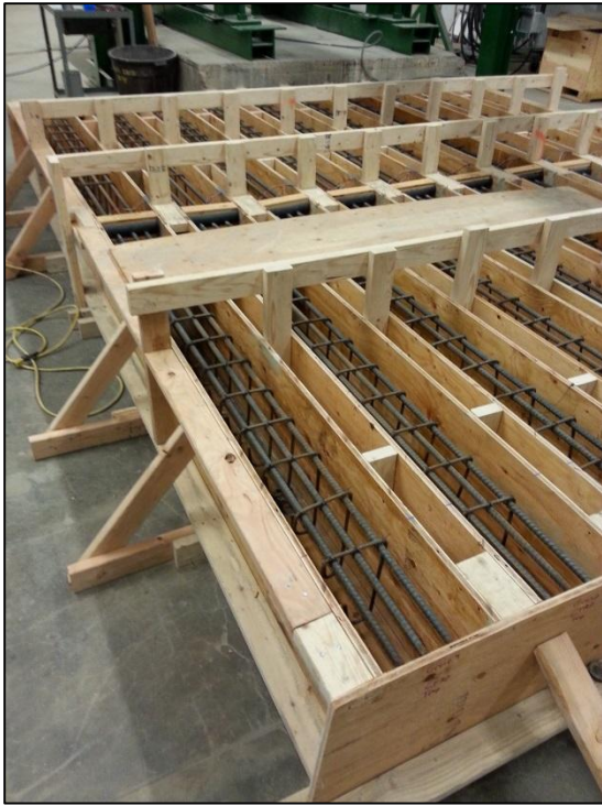
Figure 3.11 Braced plywood and lumber form-work
