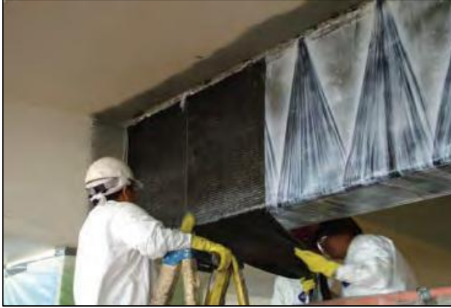
Figure 2.4 CFRP fabric sheet wet layup application to girder (CPS Construction Group 2011)
