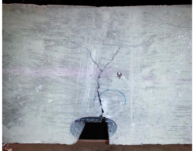
Figure 4.5 Large flexural cracking occurring immediately after fracture of second rebar in beams 2 and 3
