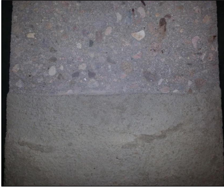
Figure 3.15 Concrete surface, top) removed laitance layer exposing aggregate, bottom) concrete surface left by finishing of wet concrete
