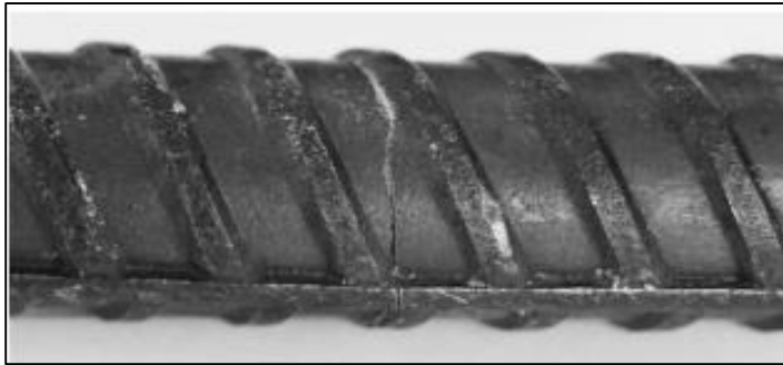
Figure 2.5 Fatigue crack in rebar with initiation at intersection of longitudinal and transverse ribs. (Derkowski 2006)
