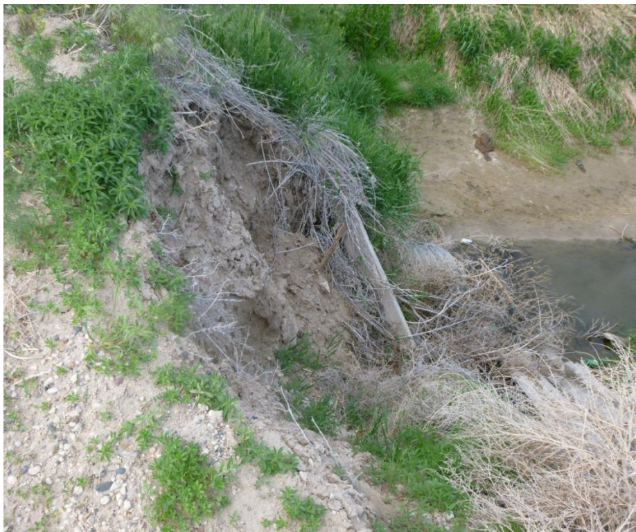
Figure 25: Example of Scour Condition State 3
