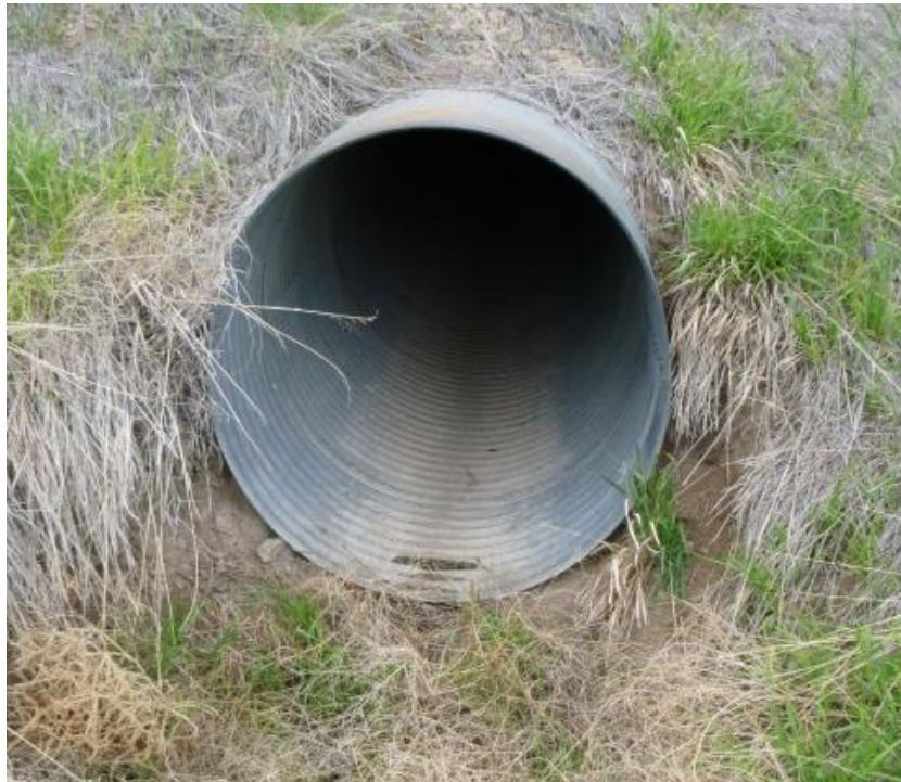
Figure 15: Example of Cracking/Corrosion State 1
