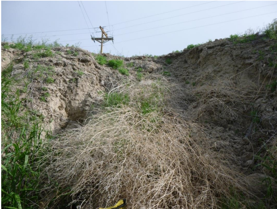
Figure 24: Example of Scour Condition State 3
