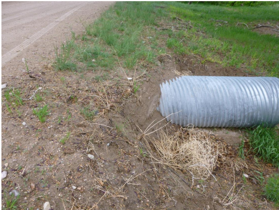
Figure 23: Example of Scour Condition State 2
