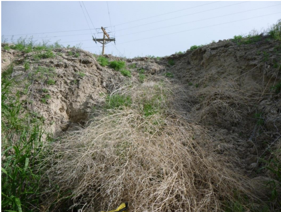
Figure 3.5 Scour Condition State 3
