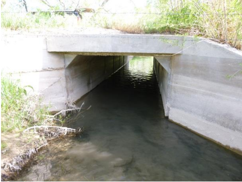
Figure 2.6 Concrete Box Culvert
