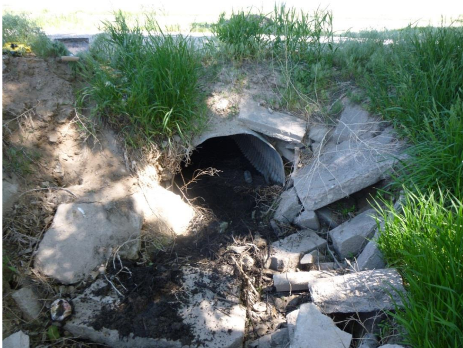
Figure 10: Example of 25% Debris
