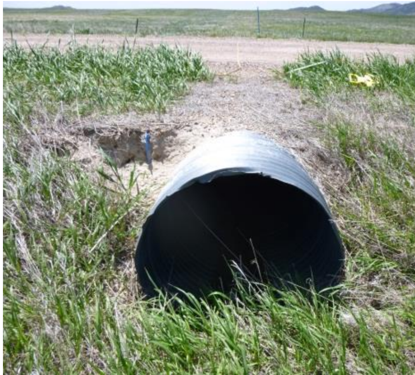
Figure 20: Example of Scour Condition State 1
