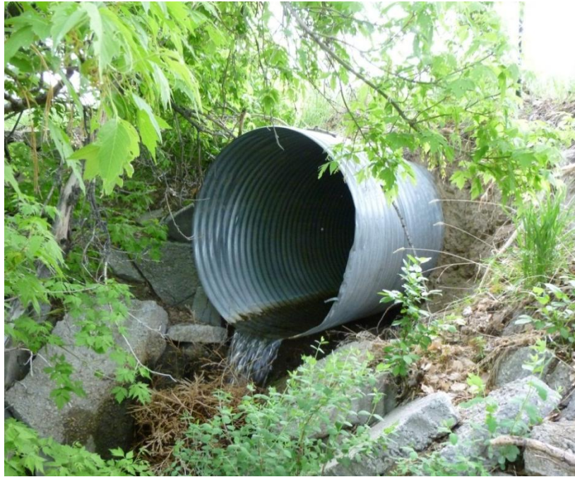
Figure 14: Example of Cracking/Corrosion State 1
