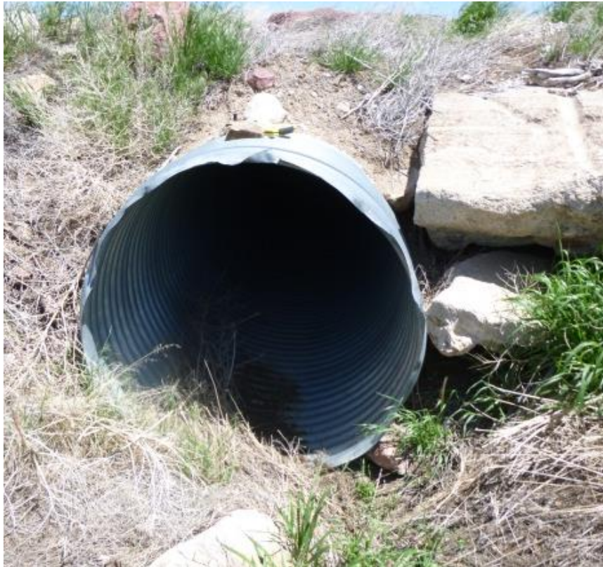
Figure 26: Example of Settlement/Deformation State 1
