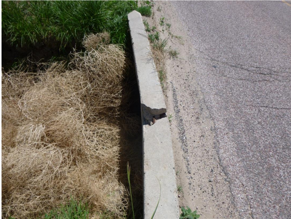
Figure 9: Concrete Retaining Wall – 3
