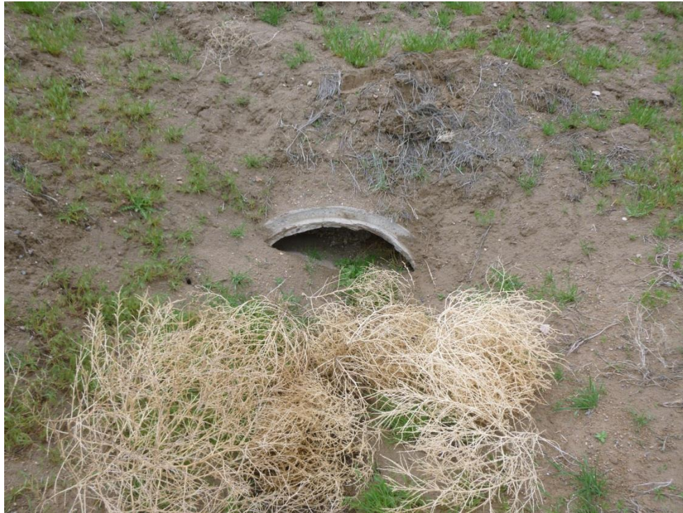
Figure 12: Example of 75% Debris
