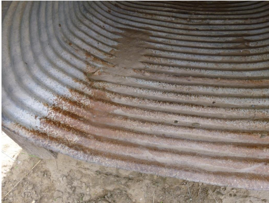
Figure 16: Example of Cracking/Corrosion State 2
