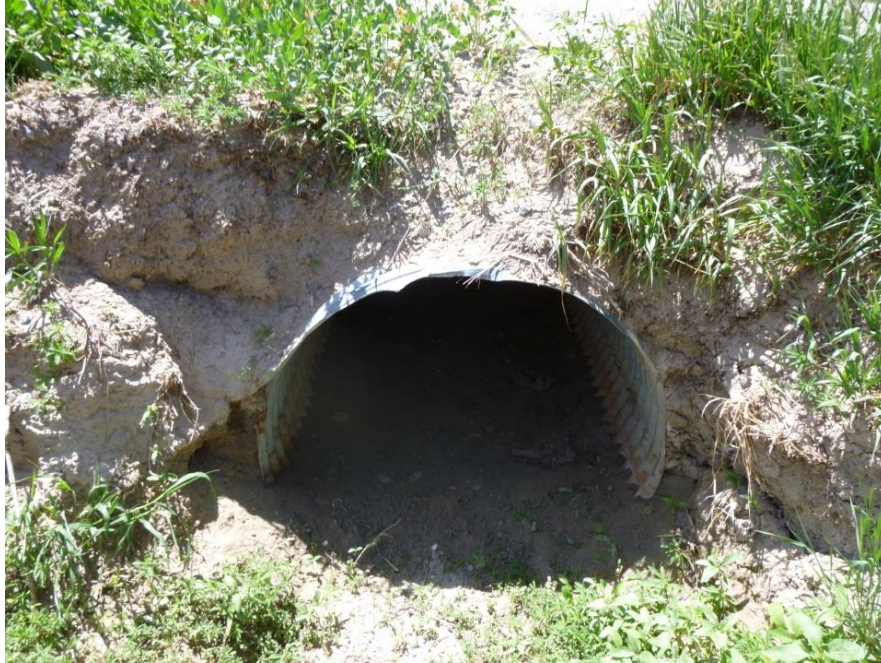
Figure 9: Example of 10% Debris
