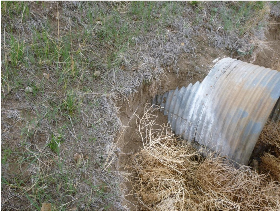
Figure 22: Example of Scour Condition State 2
