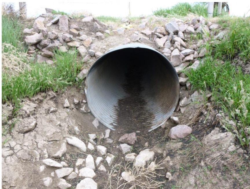
Figure 27: Example of Settlement/Deformation State 1
