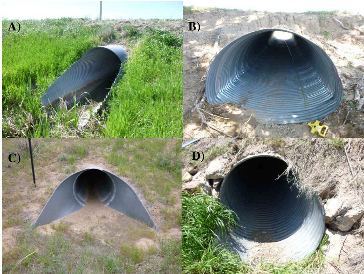
Figure 3.3 A) Open Sloped. B) Open. C) Open w/ Flared End Section. D) Open Cutback.
