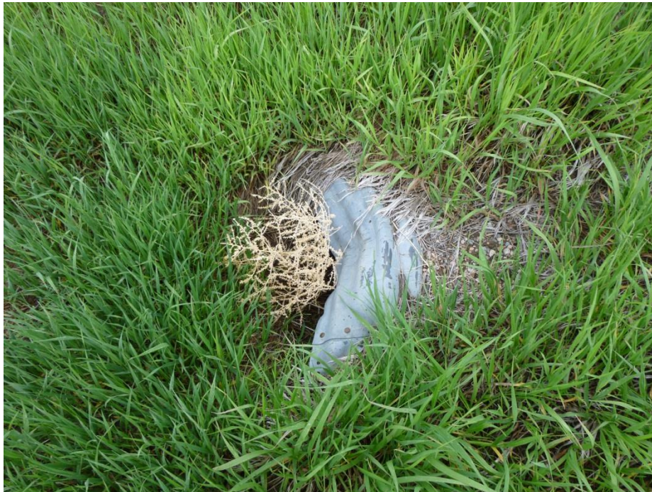
Figure 29: Example of Settlement/Deformation State 2
