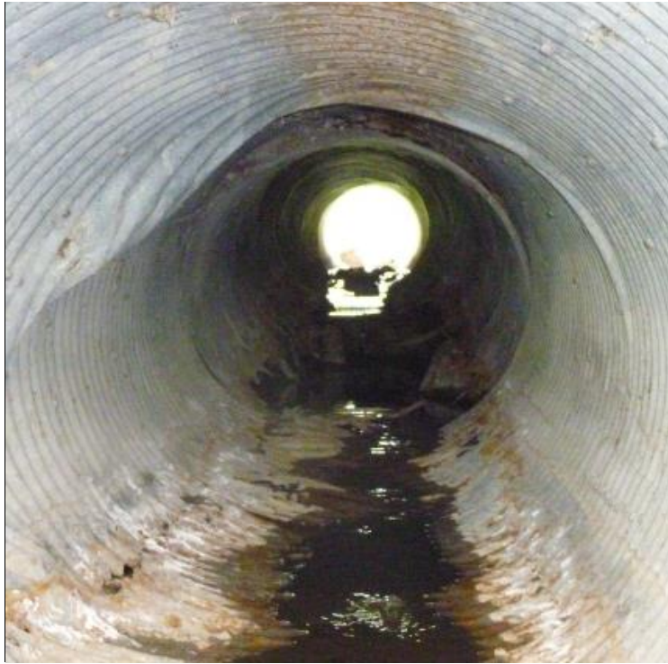
Figure 30: Example of Settlement/Deformation State 3
