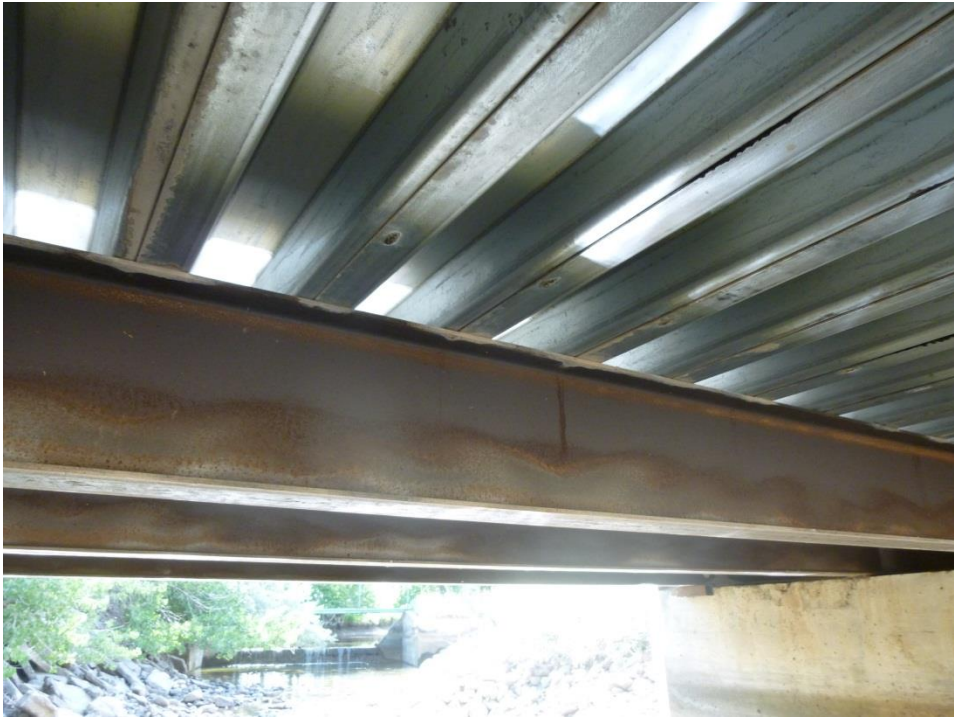
Figure 2: Steel Girder – 7
