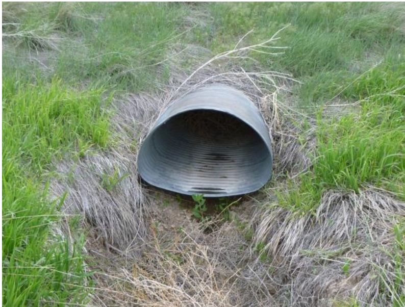
Figure 2.5 Pipe Arch Shape Culvert
