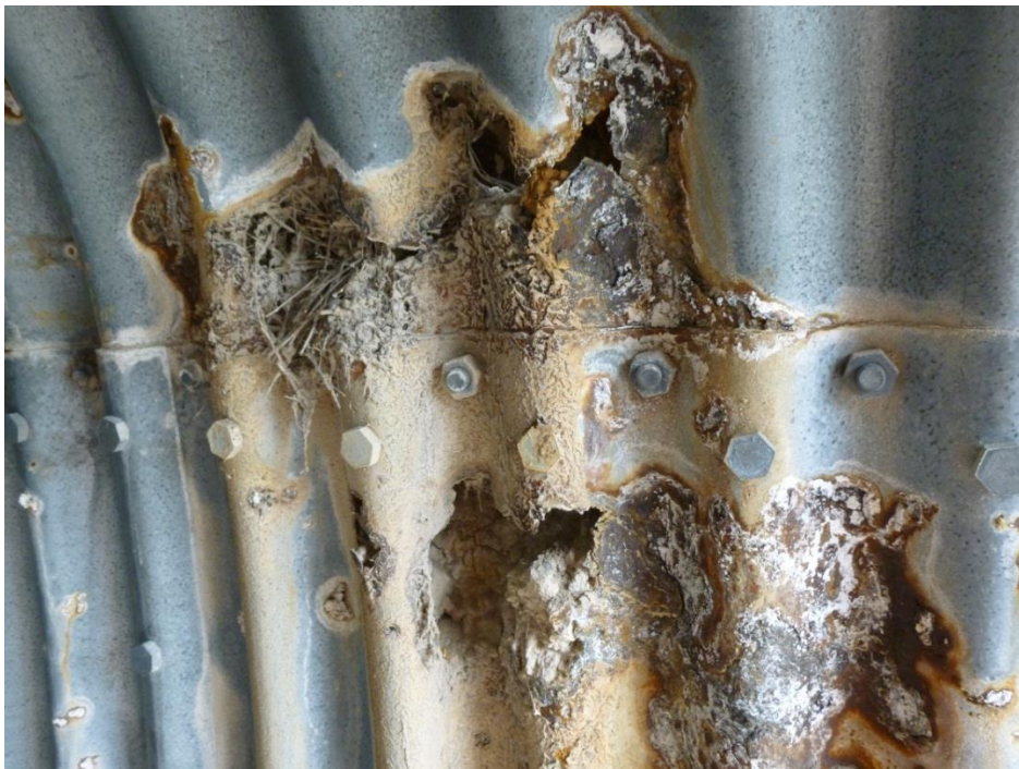
Figure 3.4 Cracking/Corrosion State 3
