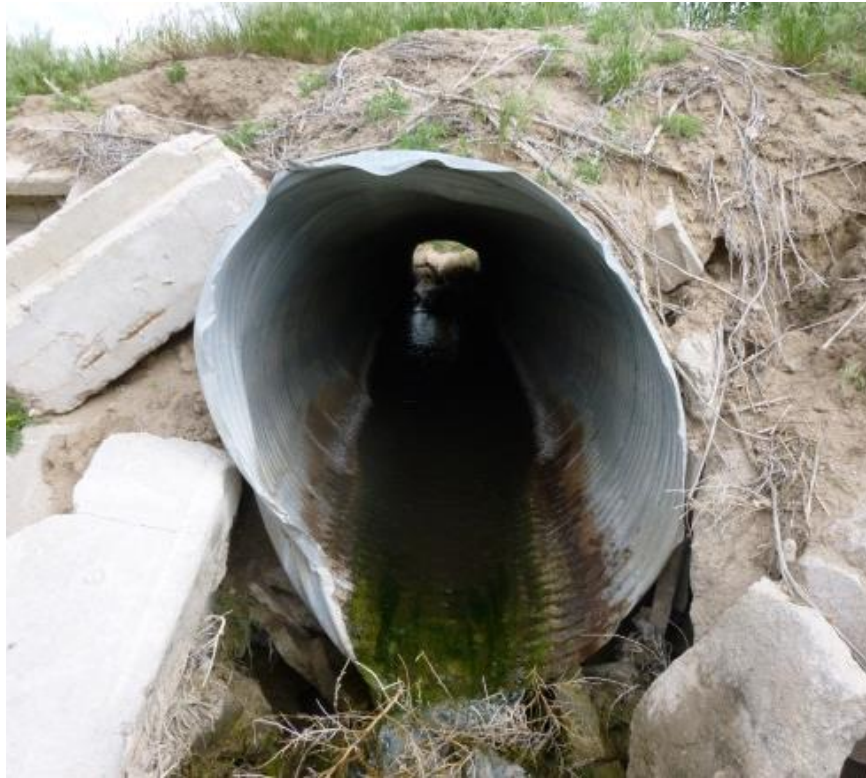
Figure 28: Example of Settlement/Deformation State 2
