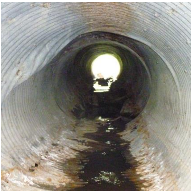
Figure 3.6 Settlement/Deformation State 3
