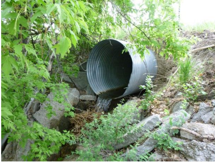
Figure 2.4 Circular Shape Culvert
