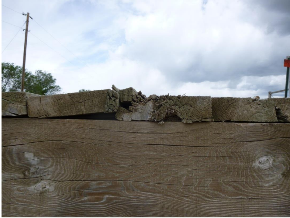
Figure 5: Timber Deck Structure – 5
