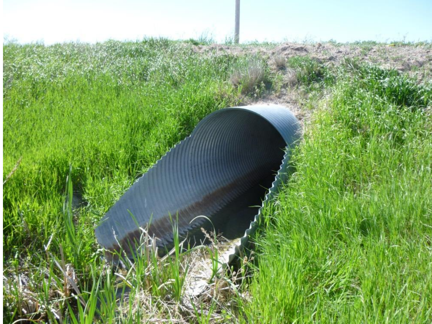
Figure 6: Open Sloped Inlet/Outlet
