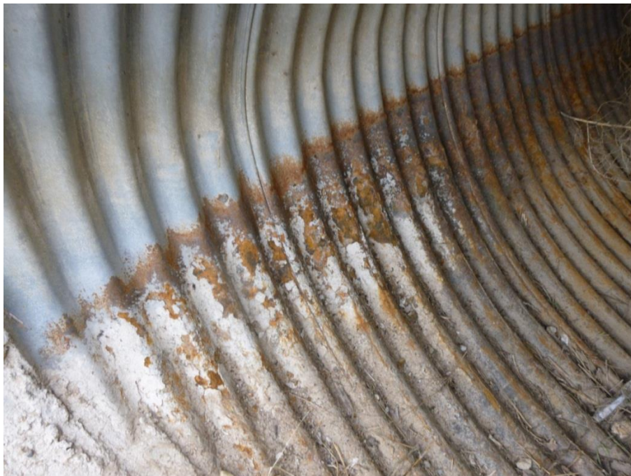
Figure 17: Example of Cracking/Corrosion State 2
