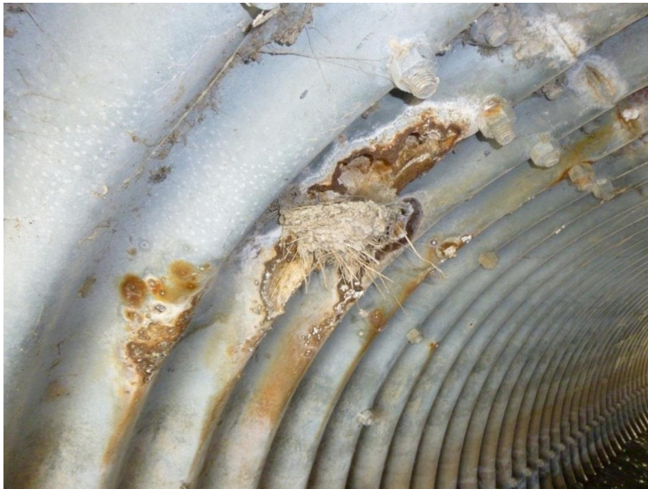
Figure 19: Example of Cracking/Corrosion State 3
