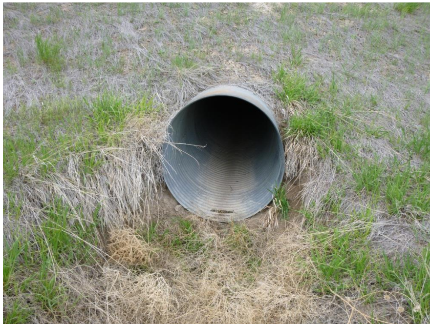
Figure 21: Example of Scour Condition State 1
