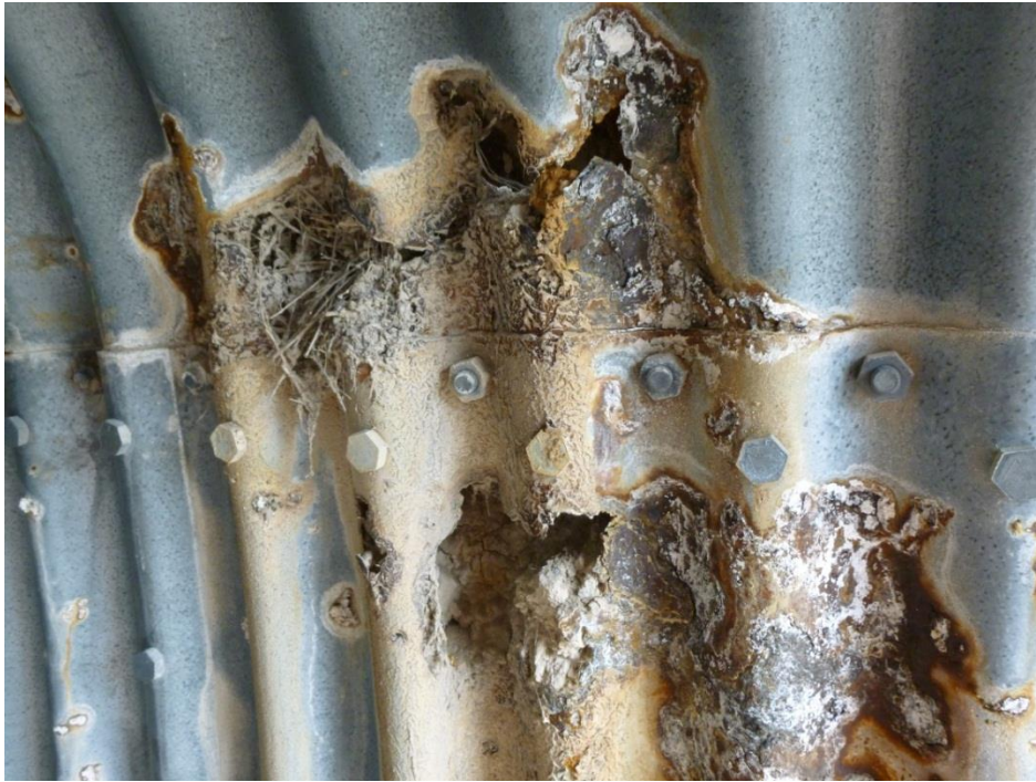
Figure 18: Example of Cracking/Corrosion State 3
