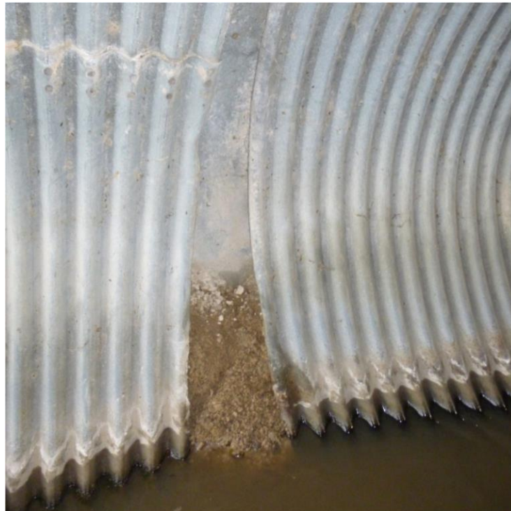
Figure 31: Example of Settlement/Deformation State 3
