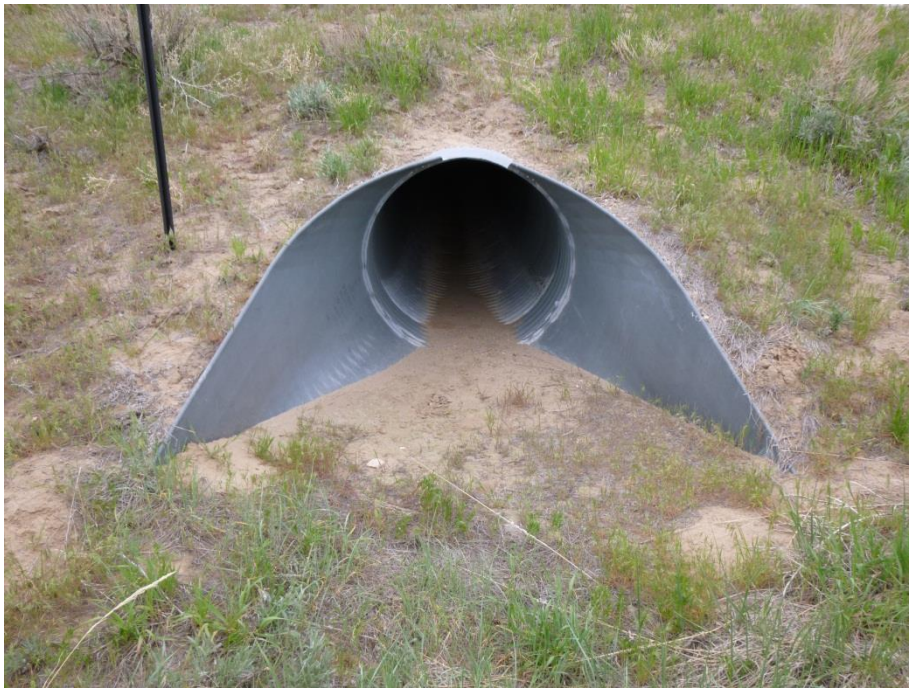
Figure 7: Inlet/Outlet with Flared End Section
