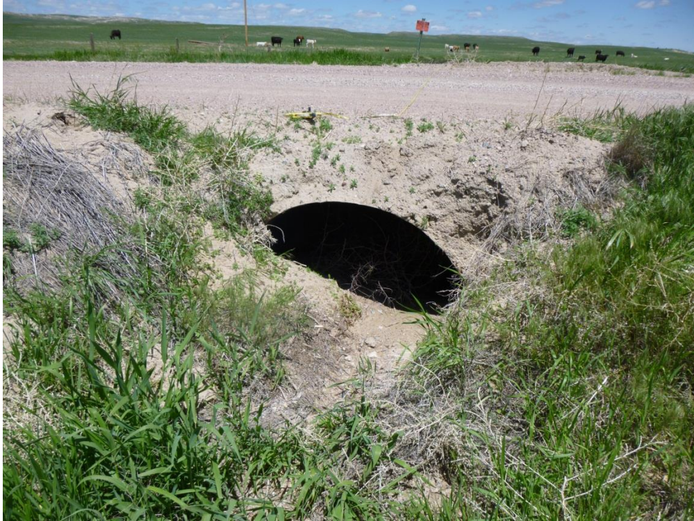
Figure 11: Example of 50% Debris
