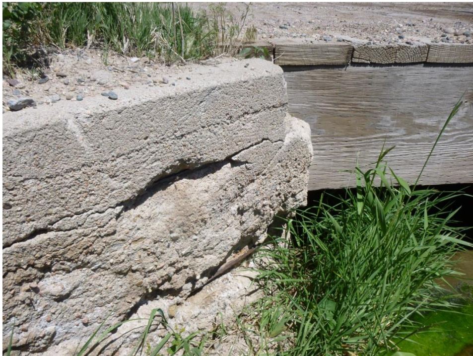
Figure 10: Concrete Wing Wall – 3
