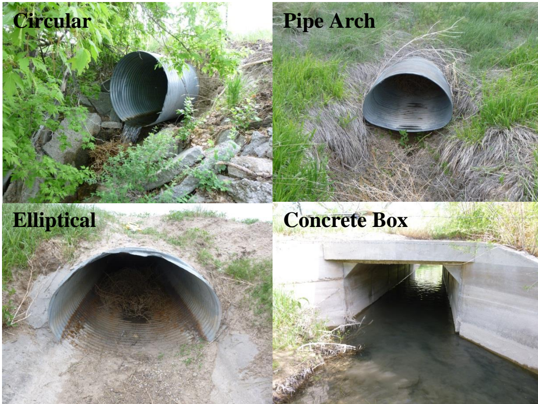
Figure 1: Barrel Shapes Commonly Found in Wyoming
