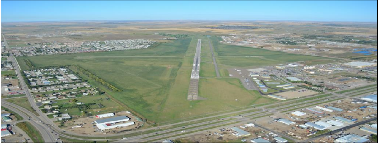
Figure 1.8 Runway at the Sloulin Field International Airport in Williston North Dakota
