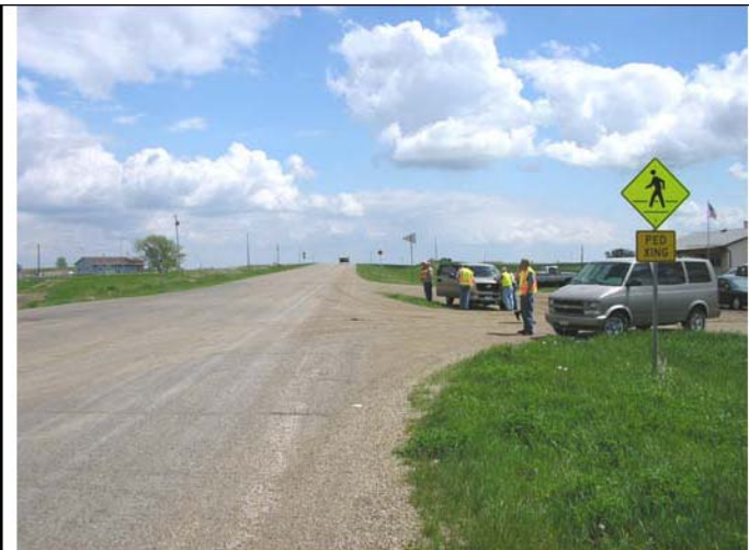
BIA 3 in Kenel, SD: Pedestrians cross BIA 3 between the residential area of Kenel (to the left in the photograph) and a grocery store (at right in the photograph). Pedestrian crossing signs have been posted on both highway approaches.
