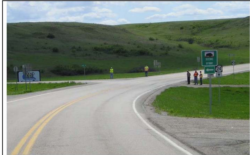
Intersection of ND24 and BIA3, looking south: No turning lane is provided for the major left-turn movement onto BIA3.
