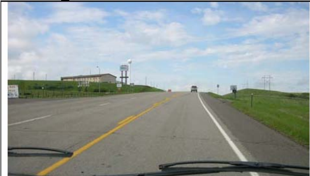
Westbound on US12 at the driveway to the Grand River Casino: No left turn lane is provided for the casino driveway at left. Westbound drivers may mistake the opposing (eastbound) left lane for a westbound turn lane.
