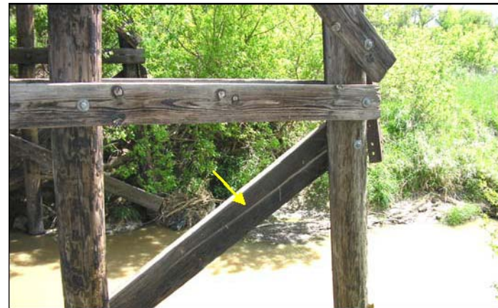
BIA 3 at Four-Mile Creek Bridge: arrow shows longitudinal crack in truss
