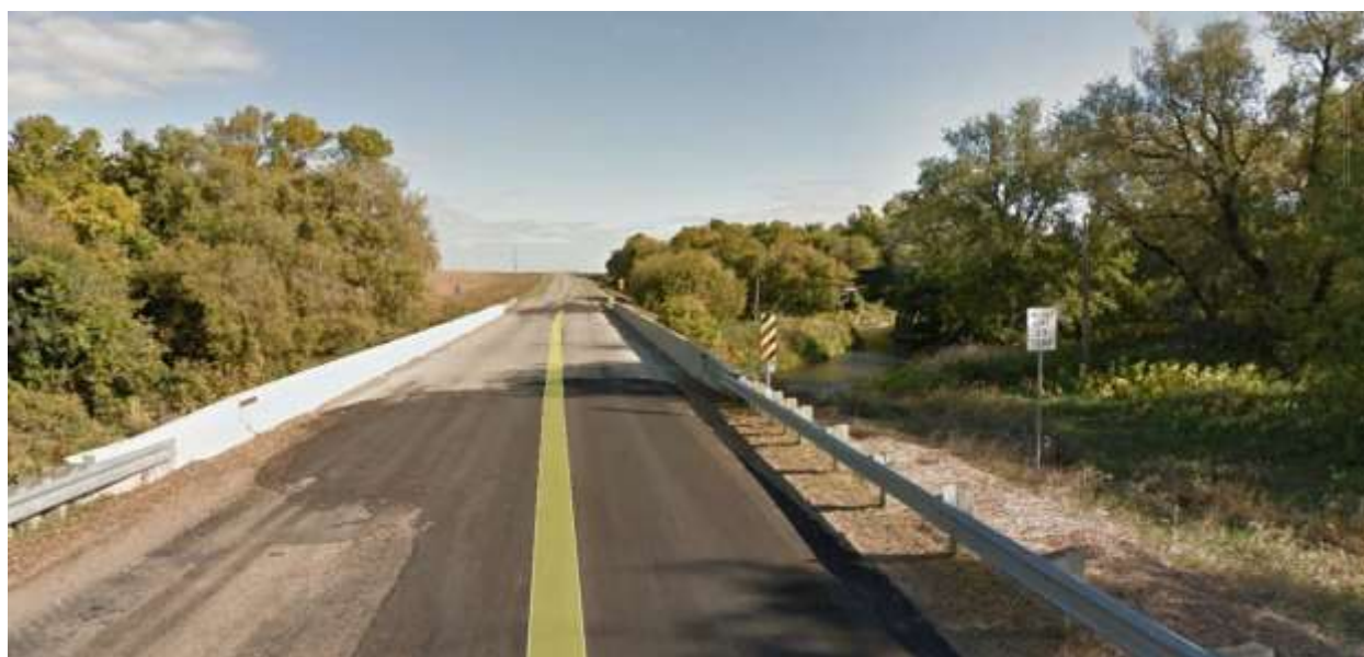
Figure 25: Existing Posted Bridge – North of Portland, ND.
